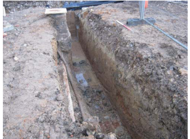
DP 4. Eastern part of the foundation trench. Looking north-east.
