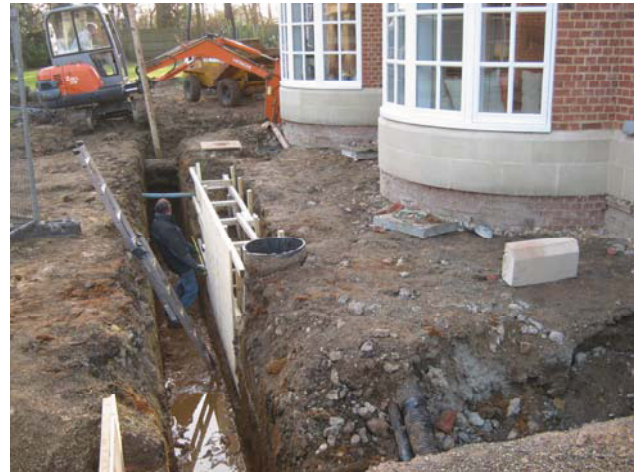
DP 2. Groundworks for new rear extension to the house. Looking south-south-west.
