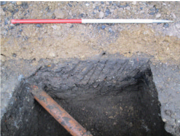
DP 5. Northern foundation trench. Sample section 1. Looking south-east.
