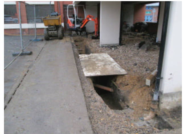
DP 6. Eastern foundation trench. Looking south-south-east.
