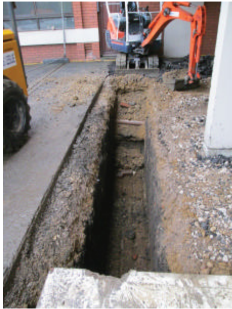
DP 7. Eastern foundation trench. Looking south-east.
