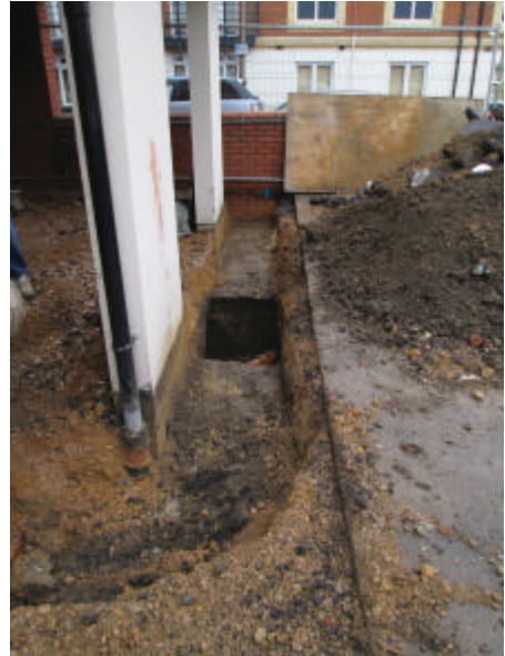
DP 4. Northern foundation trench. Looking south-west.
