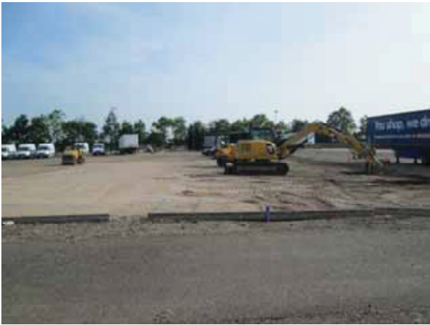
1 General view of the site looking north-east
