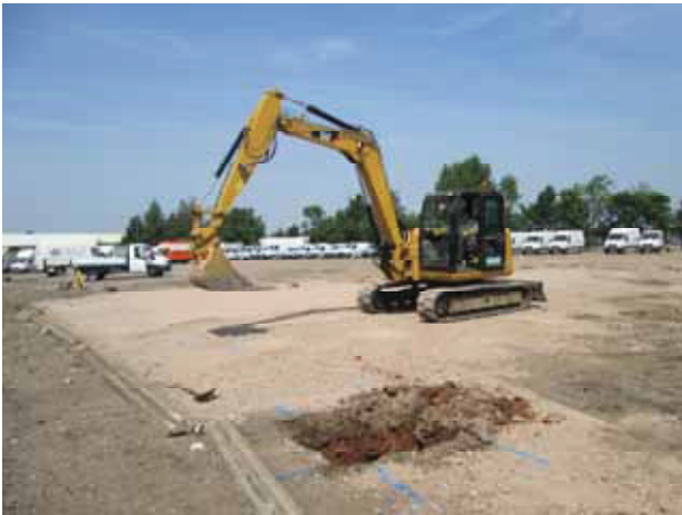
3 View of the site looking north-west
