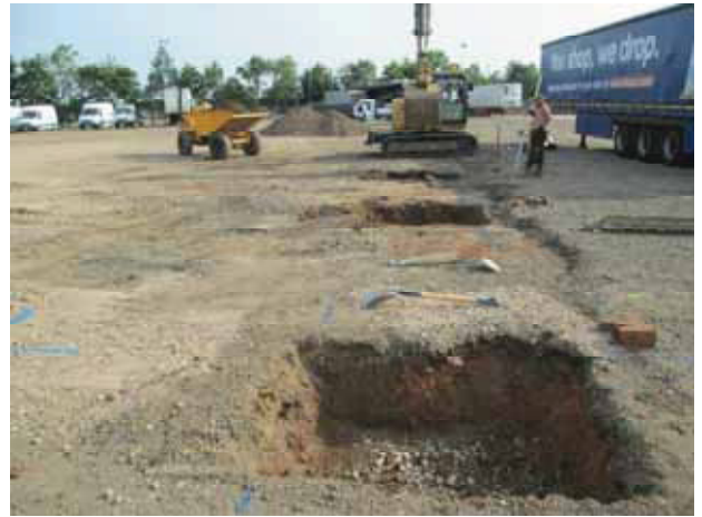
2 View of site looking north-east showing row of test pits
