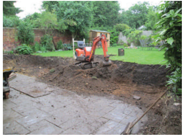
DP 2. Ground reduction. Looking north.
