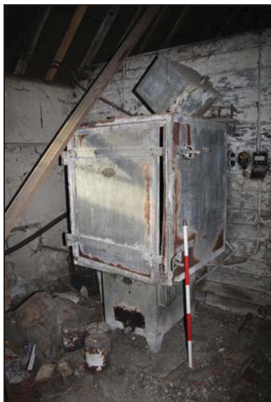
DP 35 Electric steriliser in Bay 2 (Range 2), taken from the north-west
