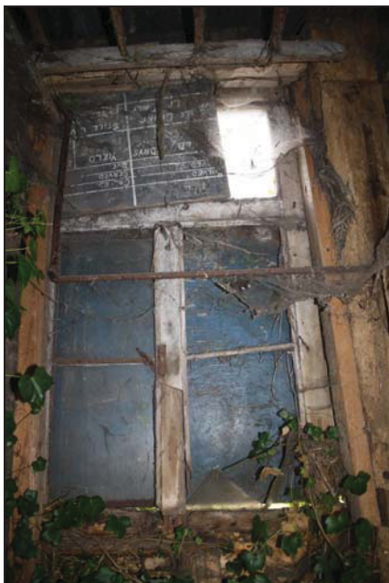
Transom and mullion window on the north side of Bay 2 (Range 1), taken from the south
