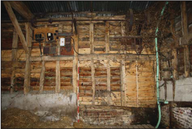
DP 43 Reused early window transom on the north side of Bay 3 (Range 1), taken from the south-east
