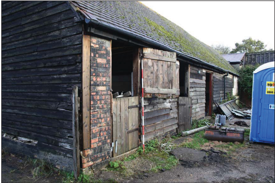
Plate 4 East elevation of Range 2, taken from the south (DP 9)
