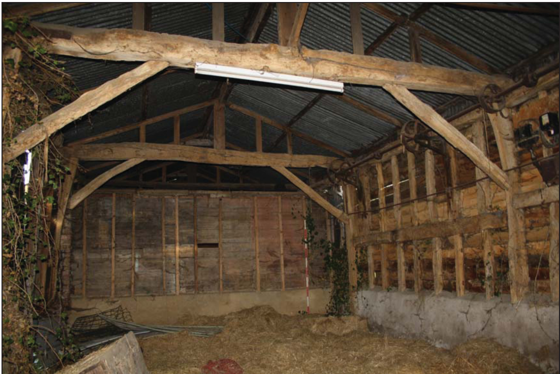
Plate 2 Eastern bays of Range 1, taken from the east (DP 32)
