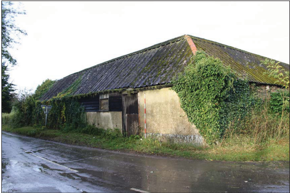
Plate 8 East elevation of Range 4, taken from the north-east (DP 3)
