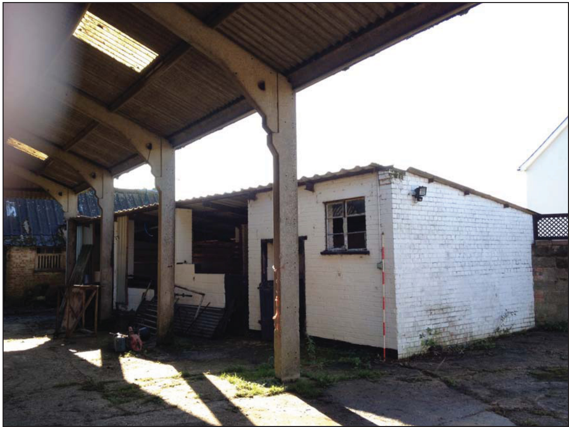
Plate 11 North and west elevation of Range 6, taken from the north-west (DP 13)
