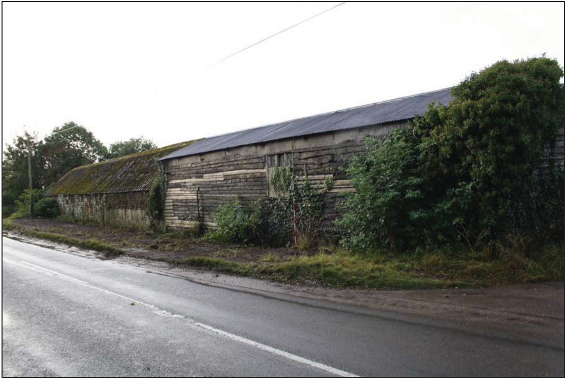
Plate 1 North elevation of Ranges 1 and 3, taken from the north-west (DP 3)
