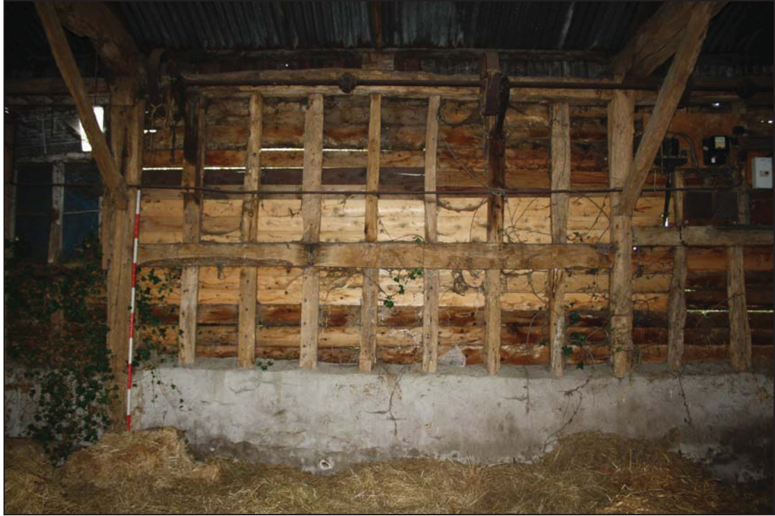
Plate 3 North side of Bay 3 (Range 1), taken from the south (DP 42)
