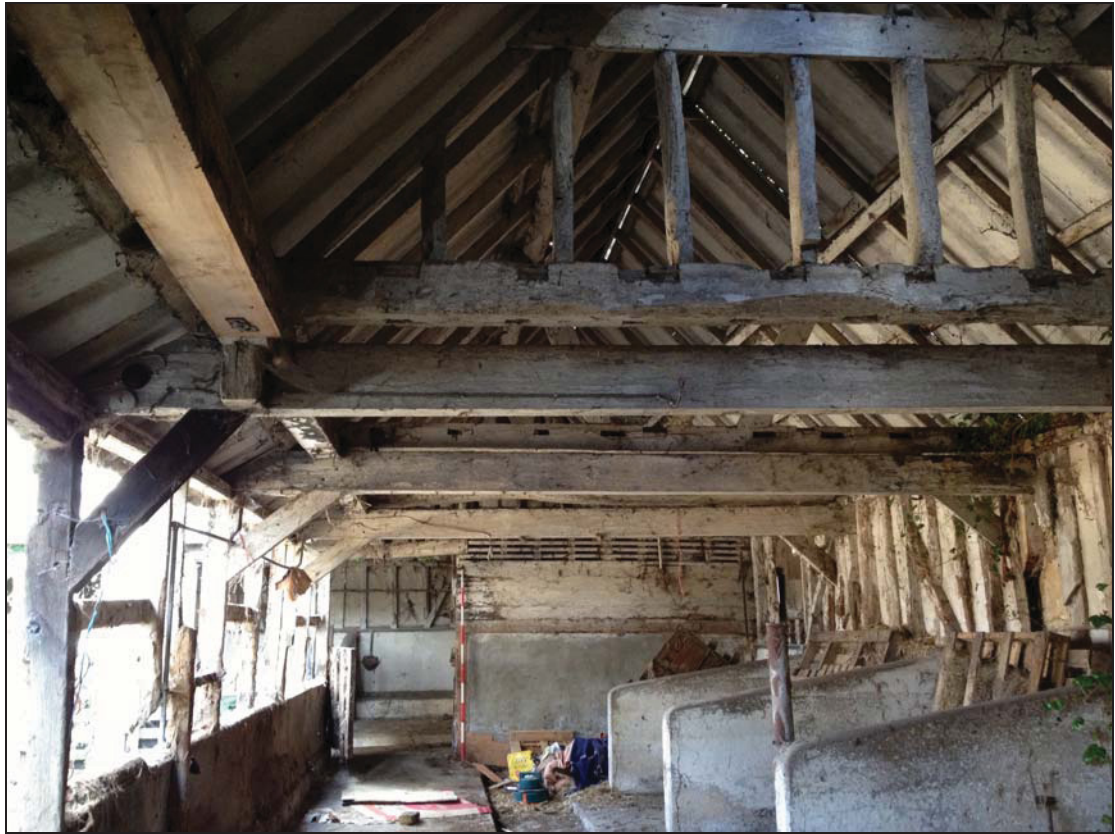
Plate 9 North end of Range 4, taken from the south (DP 23)
