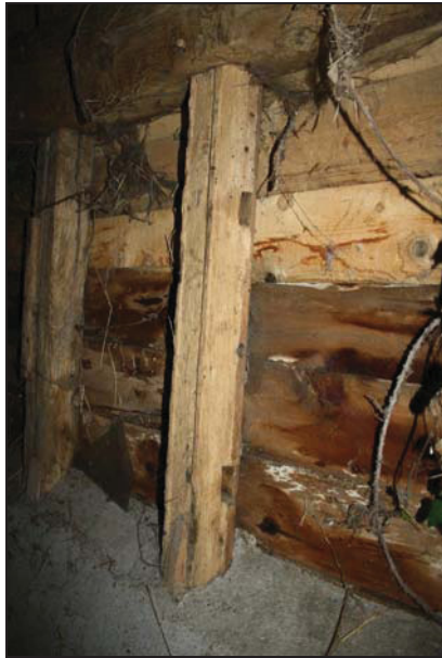
DP 43 Reused early window transom on the north side of Bay 3 (Range 1), taken from the south-east
