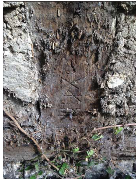
DP 28 Assembly mark on a stud on the south side of Bay 8 (Range 3), taken from the south
