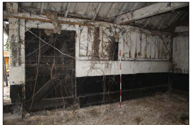
DP 48 South side of Bays 1 and 2 (Range 3), taken from the north
