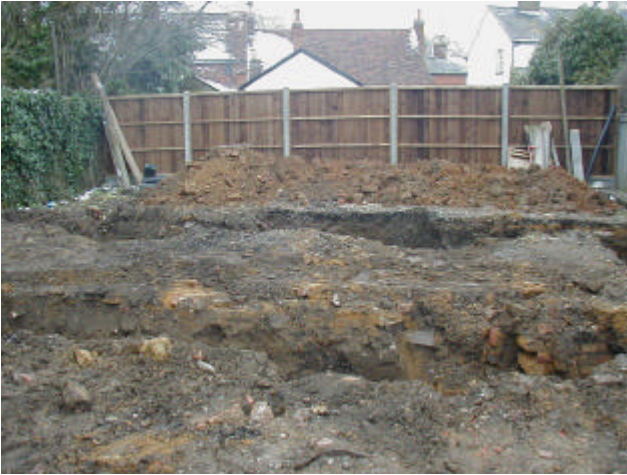
DP 1. Western part of the site. Looking west.
