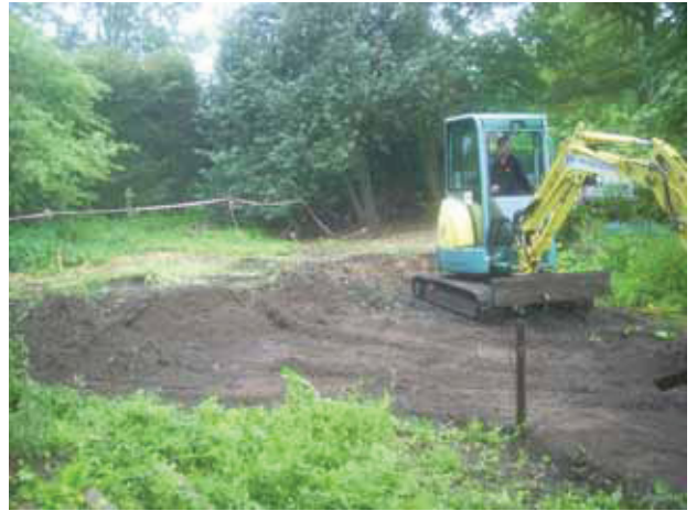
2 Soil stripping in progress
