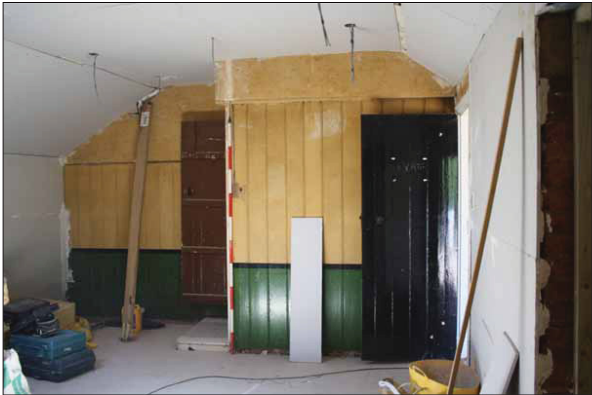
Plate 5 West end of the south-east range (Room GF02) showing staircase and match-lined boarding to the main range, taken from the east (DP 26)
