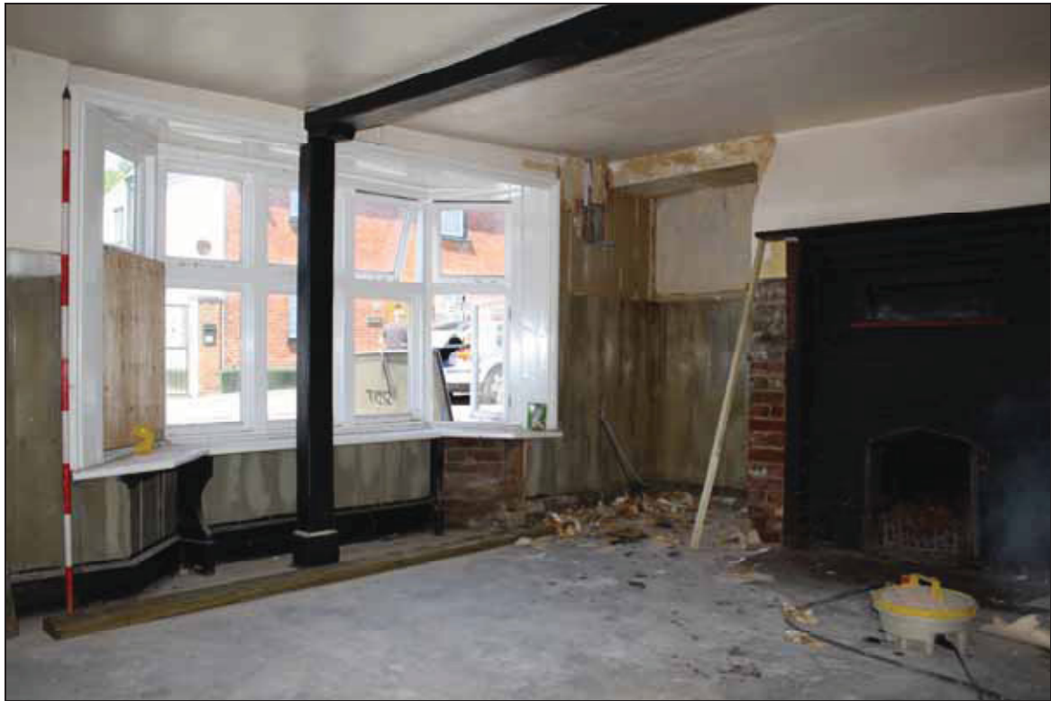
Plate 3 North end of Room GF01, taken from the south-east (DP 19)
