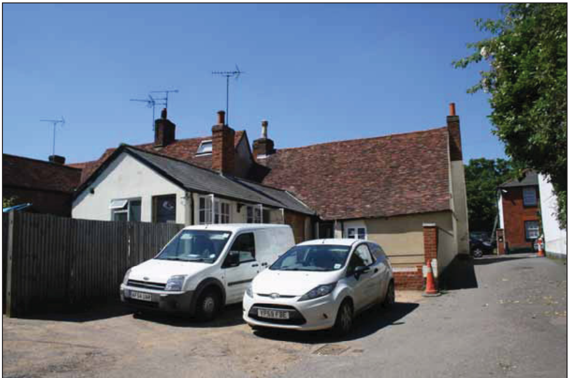
Plate 2 View of the assessment structure after the removal of the north-east range, taken from the east (DP 13)
