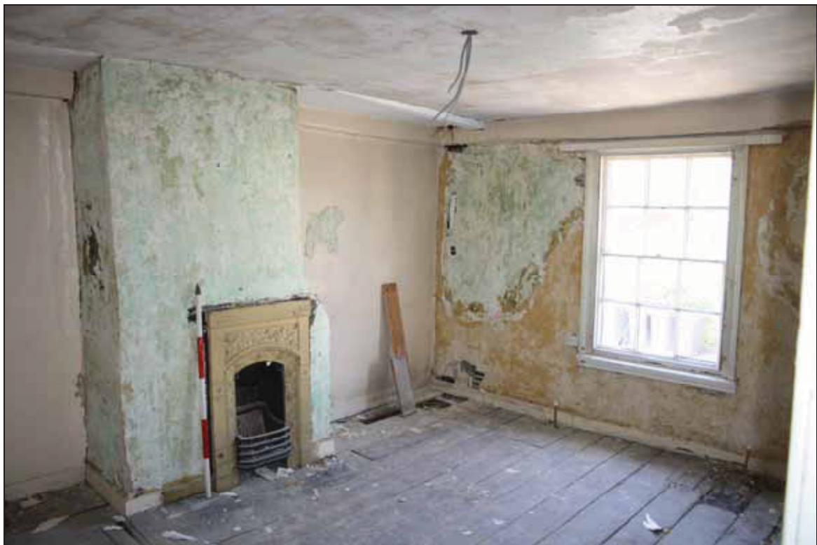
Plate 6 Room FF03, taken from the north-east (DP 35)
