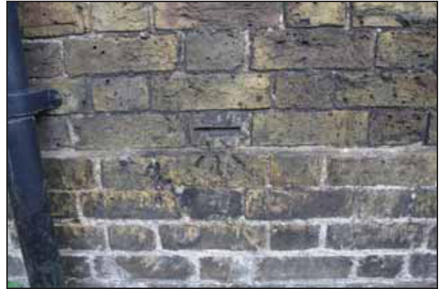
Detail of bench mark on the single storey block taken from the north
