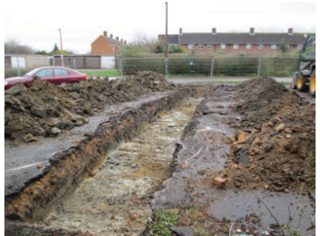
DP 6. Trench 2. Looking south-east.
