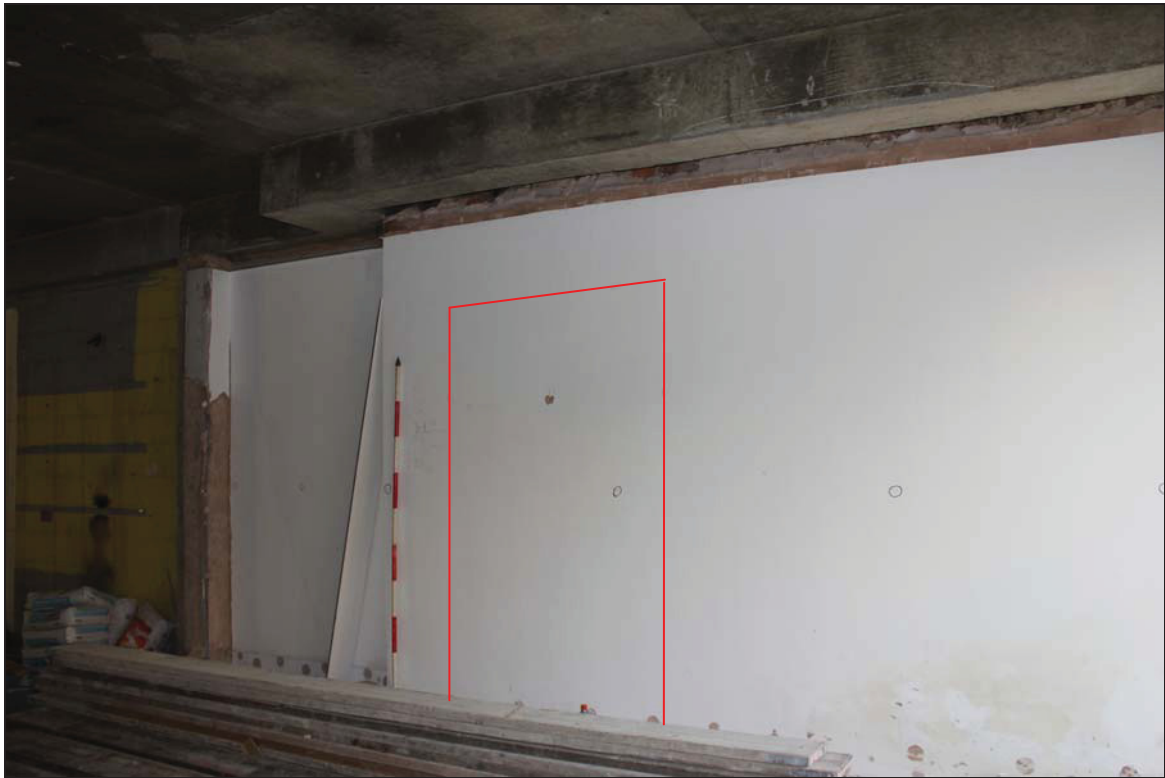
Plate 5 South wall of Room GF02 (No. 24) with position of new doorway outlined, taken from the south-west (DP 6)
