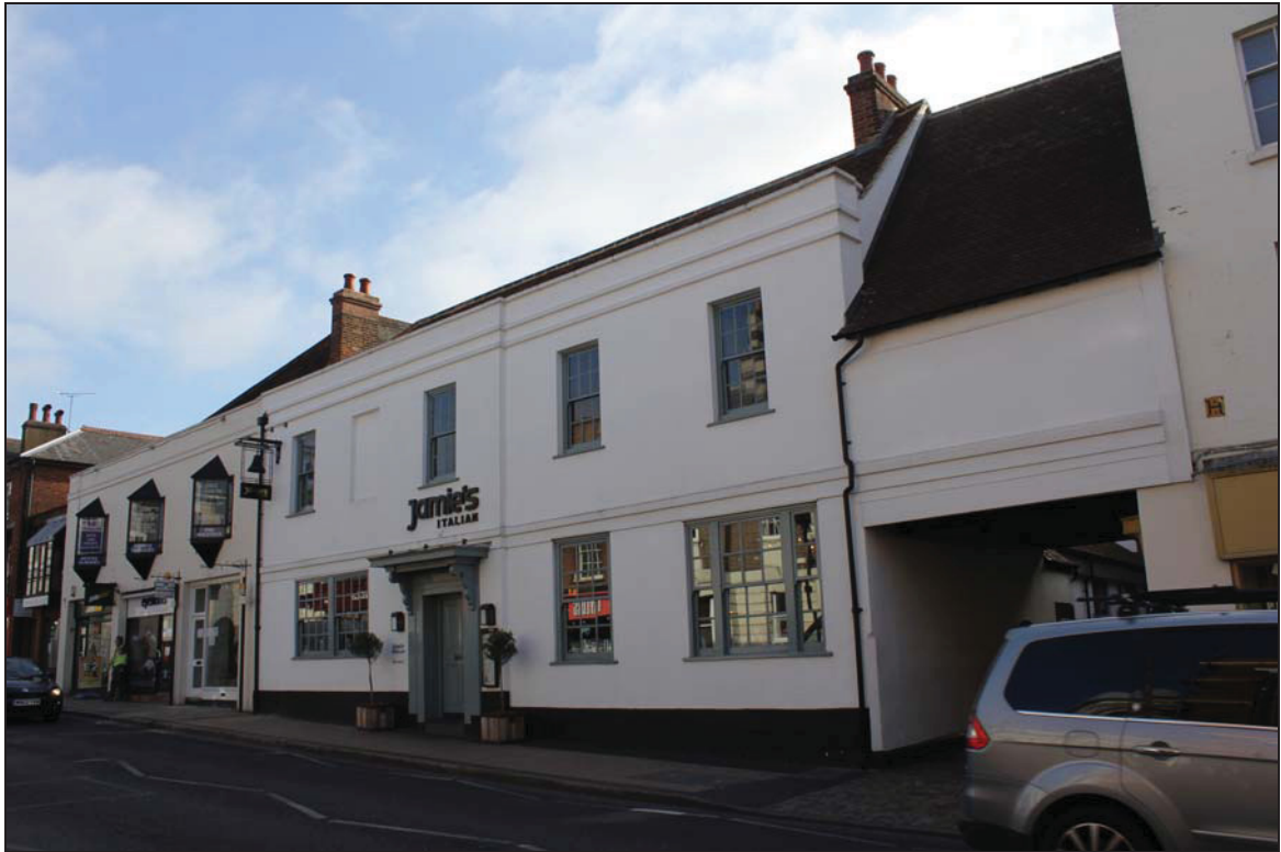
Plate 1 West street front elevation of Nos. 22 (right) and Nos. 24-26 (left), taken from the south-west (DP 12)
