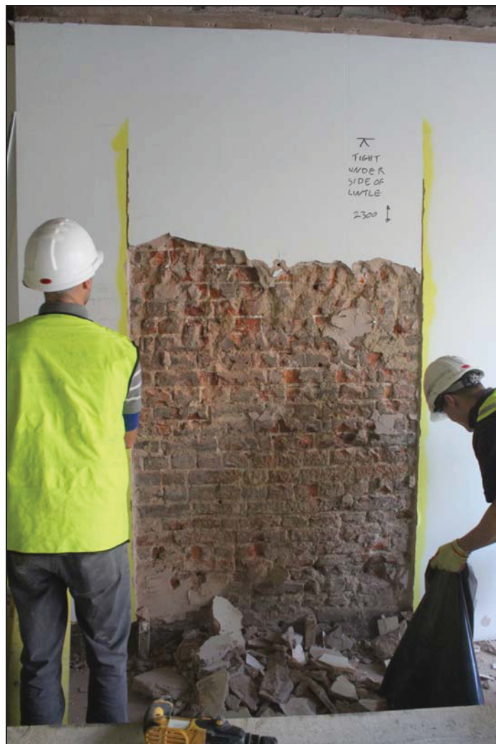
Plate 6 Brick work exposed during insertion of the new doorway, taken from the north (DP 10)
