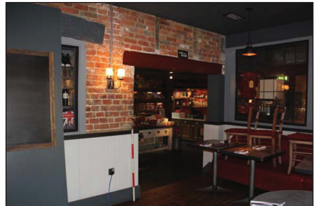
DP 4 East wall of Room GF01 (No. 22) showing further exposed brickwork with timber elements as well as recent modern fabric, taken from the north-west
