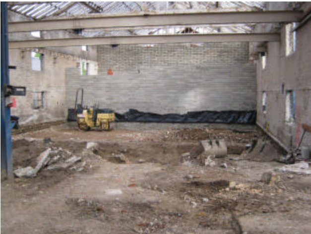
DP 11. Central/east part of the building. Looking east.
