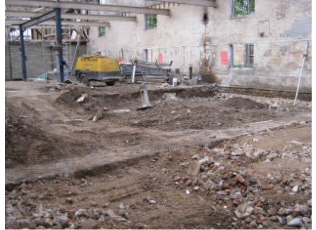
DP 8. Central part of the building. Looking north-west.
