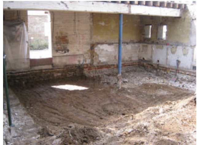
DP 12. Western end of the building. Looking south-west.
