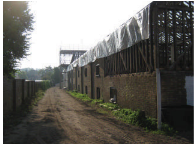
DP 2. Northern side of the building. Looking east.
