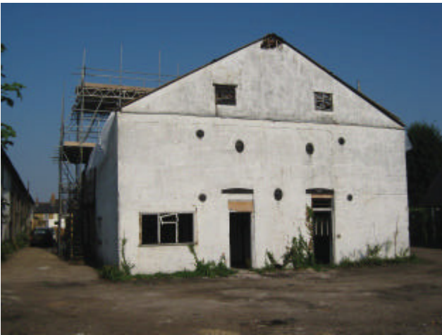
DP 3. Eastern façade of the building. Looking west.
