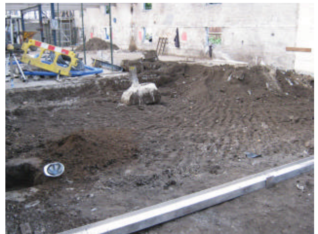
DP 6. Eastern part of the building. Looking north-west.
