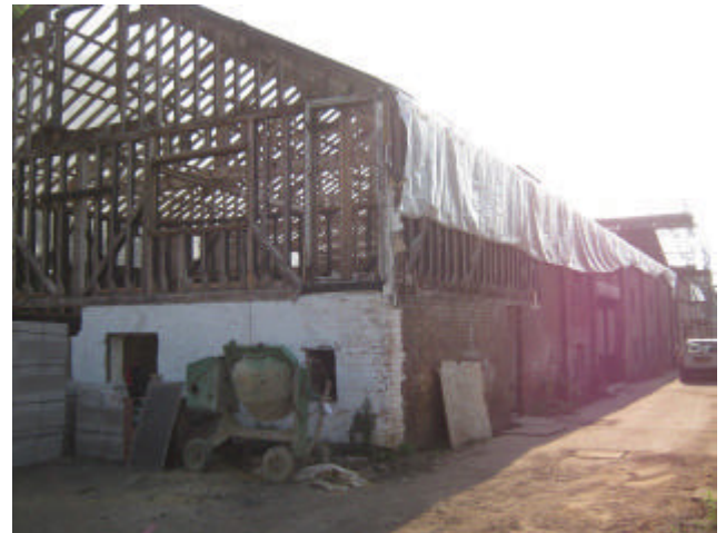
DP 4. Southern side of the building. Looking north-east.
