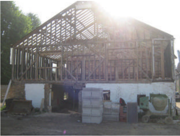
DP 1. Northern Maltings, western façade. Looking east-north-east.
