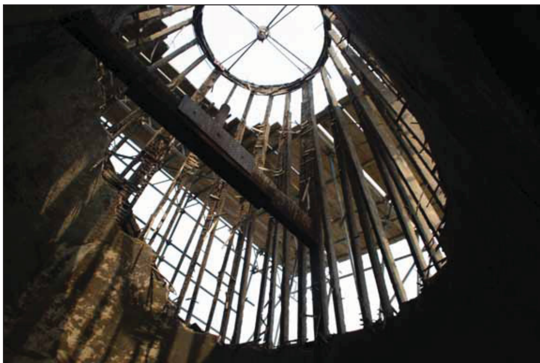
Plate 12 Looking into northern kiln with supporting cross beam for cowl now removed, taken from the south-east (DP 47)
