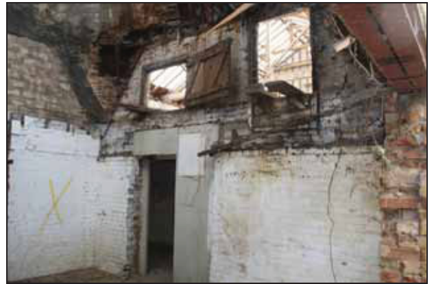
Southern kiln with upper joists removed and small doors and hatches giving access to the dispatch end of the building, taken from the south-west
