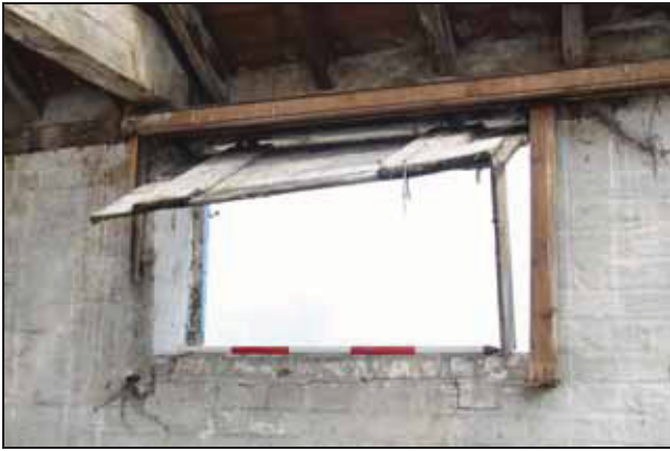
Aperture with top-hung shutter, north elevation, dispatch office, first floor, taken from the south-east
