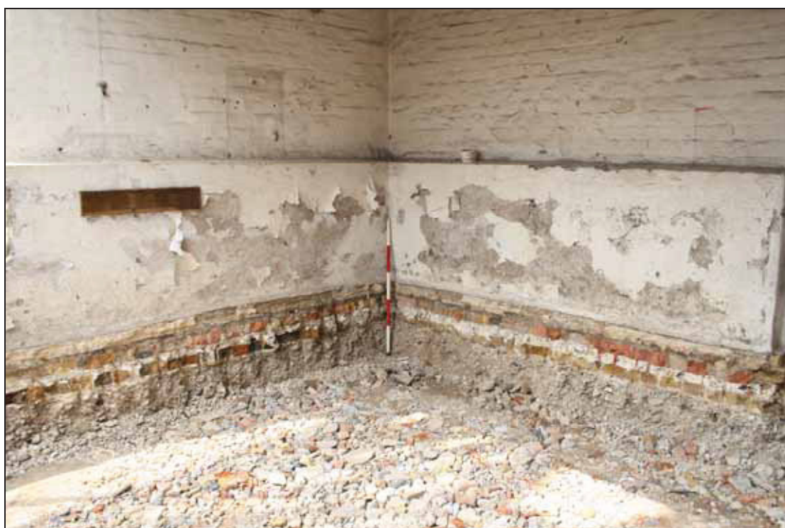
Plate 6 Remains of a steeping tank, western end of the maltings, taken from the south-east (DP 63)
