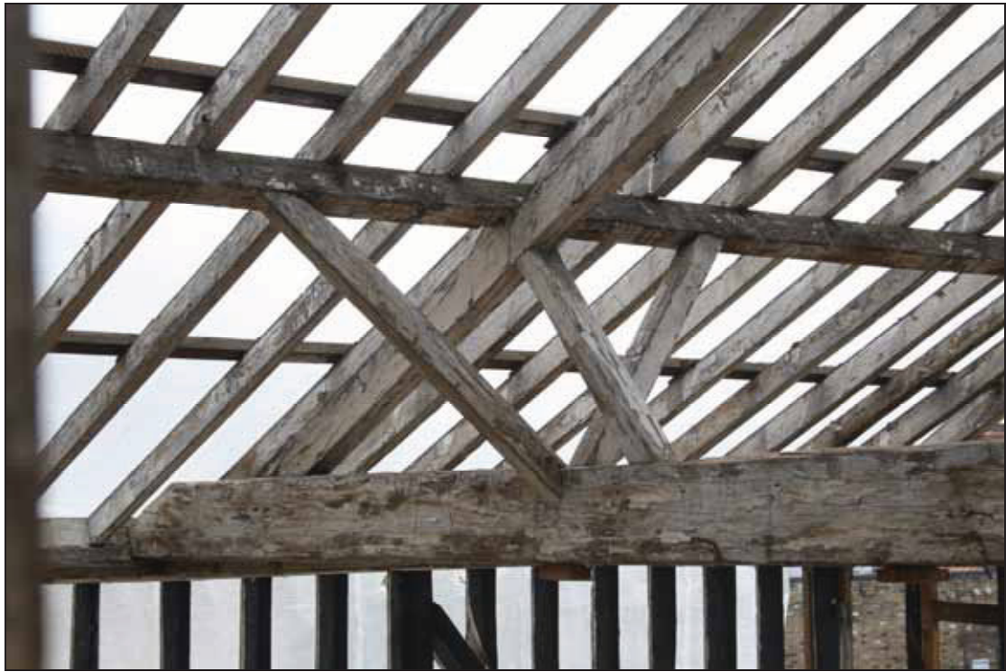
Plate 8 Roof structure with additional raking struts supporting the purlins from the tie-beam, taken from the north-east (DP 68)
