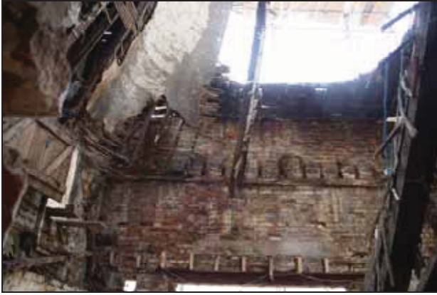
Partially demolished southern kiln with floor joists removed, taken from the north-east
