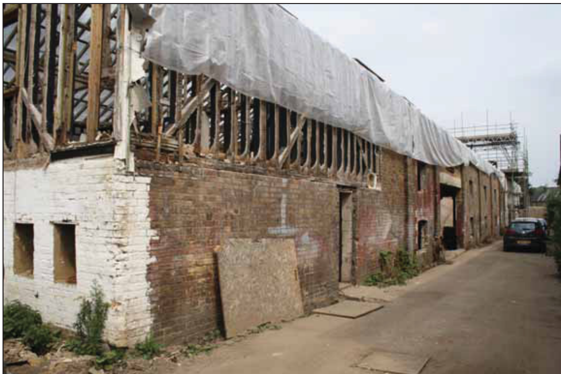
Plate 2 Timber-framed upper section, western end of the south elevation, taken from the south-west (DP 11)
