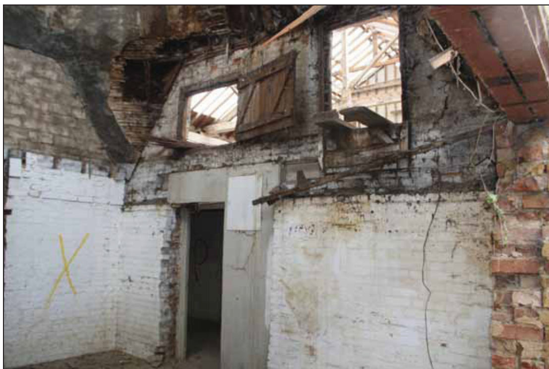
Plate 11 Southern kiln with upper joists removed and small doors and hatches giving access to the dispatch end of the building, taken from the south-west (DP26)
