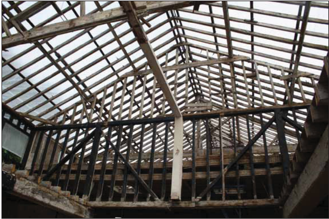
Plate 7 Timber-framed partition between the western section and central section of the maltings, taken from the south-west (DP 65)
