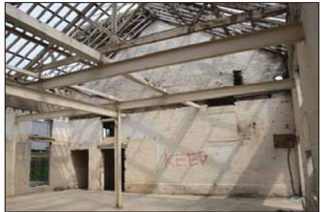
Timber structure possibly supporting a crane, dispatch office, first floor, taken from the north-west
