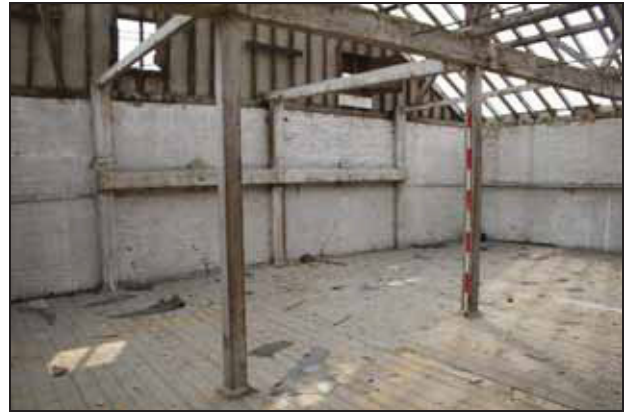
Timber structure possibly supporting a crane, dispatch office, first floor, taken from the north-west
