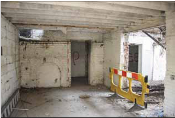
Ceiling joists supporting upper floor, dispatch office, ground floor, taken from the east
