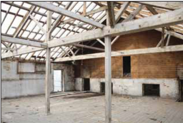
Partially demolished southern kiln with floor joists removed, taken from the north-east
