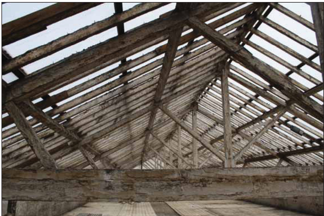
Plate 10 Highly consistent roof structure, formed of identical king-post trusses, taken from the north-west (DP 69)
