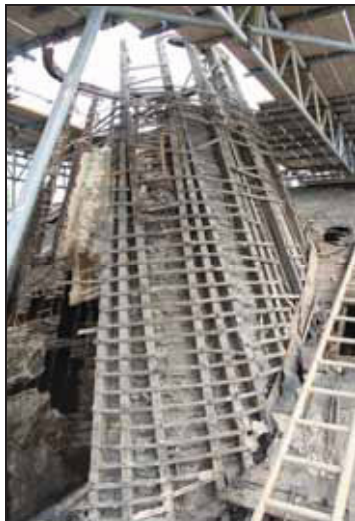
Timber framed construction of southern kiln, taken from the south-east
