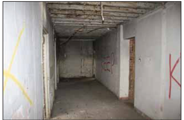
Southern kiln with upper joists removed and small doors and hatches giving access to the dispatch end of the building, taken from the south-west
