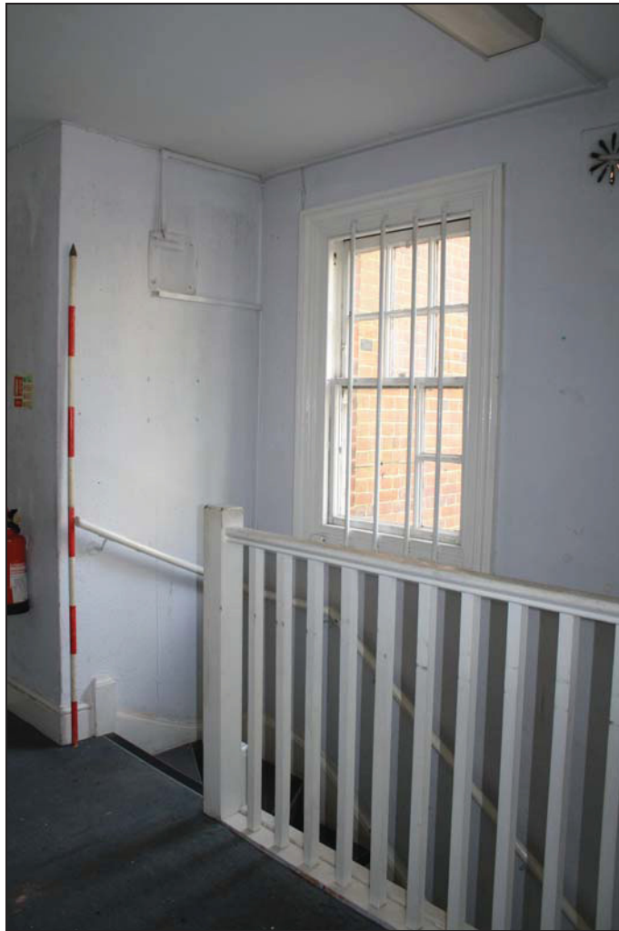
Plate 11 First floor landing of the northern staircase (Room FF01), taken from the north (DP 41)
