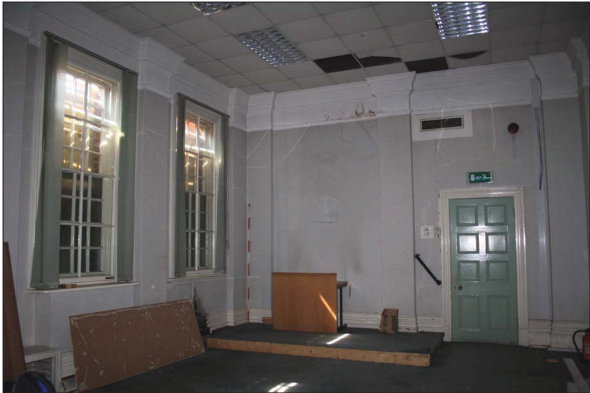
Plate 5 Court 2 (Room GF07), taken from the north (DP 21)
