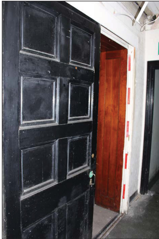
Plate 9 Studwork partition on the west side of the central bay of Building 5, taken from the east (DP 22)
