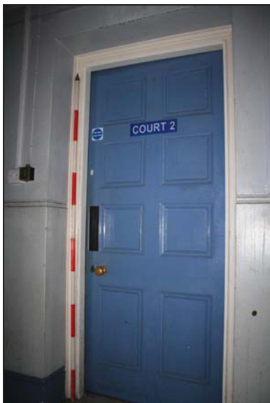
DP 23 North-east door to Room GF07 (GF04), taken from the north-west
