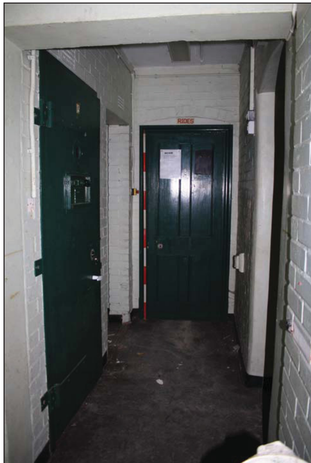
Plate 10 West cell block (Room GF15), taken from the north-west (DP 30)
