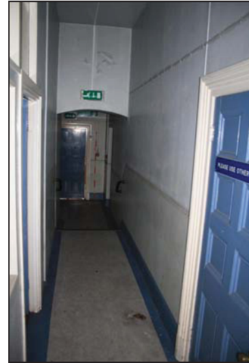
DP 20 Corridor GF04, taken from the north-west
