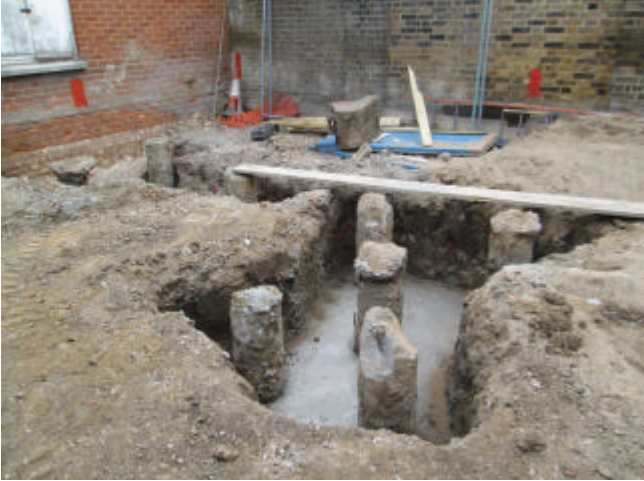
DP 13. North-eastern foundation trench. Looking north-east.
