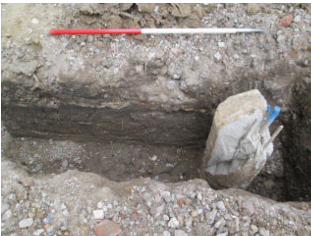
DP 11. Foundation trench in south/central part of the site. Sample section 5. Looking west-south-west.
