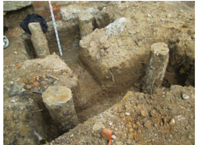
DP 8. . Foundation trenches in north-western corner. Looking north-north-west.
