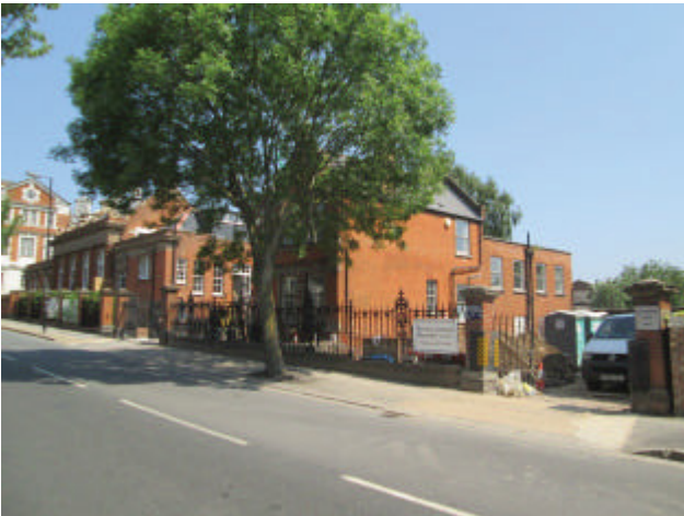
DP 1. View for the site from Winchester Street. Looking north-east.
