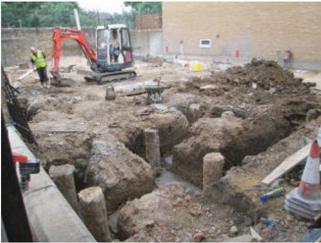
DP 7. Foundation trenches in western part of the site. Looking east.
