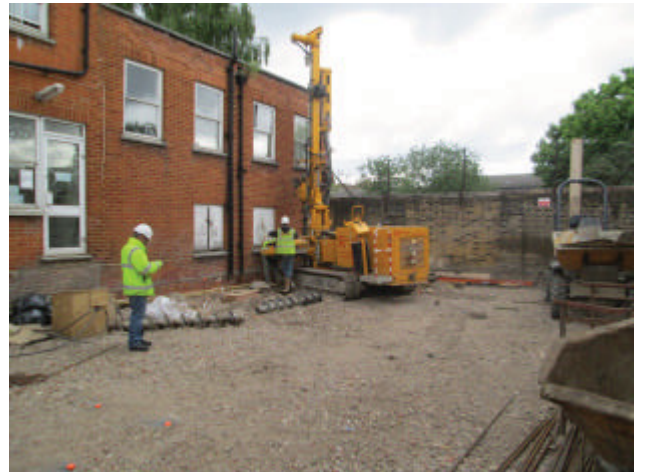
DP 2. Piling in progress. Looking north-east.
