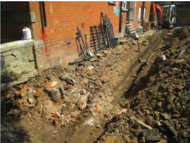
DP 3. Service trench along northern side of the site. Looking east-north-east.
