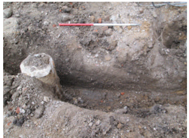
DP 12. South-eastern foundation trench. Sample section 6. Looking east-north-east.
