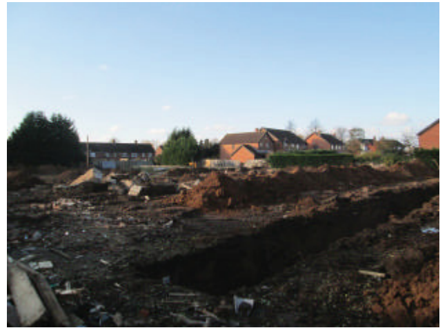
DP 2. The site. Looking north-west.
