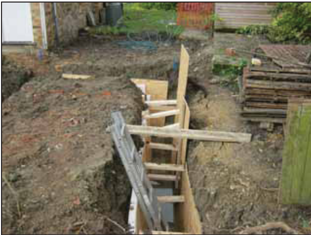
Front extension footing trench. Looking WSW.
