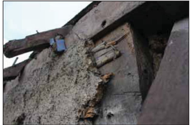
External Render over lath and plaster at the principal-post, north-west elevation, taken from the south-west
