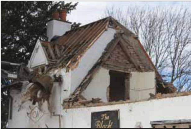
Original southern end truss to historic core against later 20 th century brick addition, taken from the north-east
