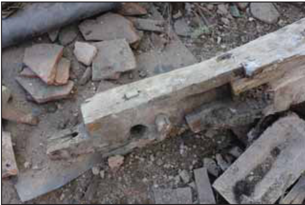
Mid-rail section showing exposed scarf joint
