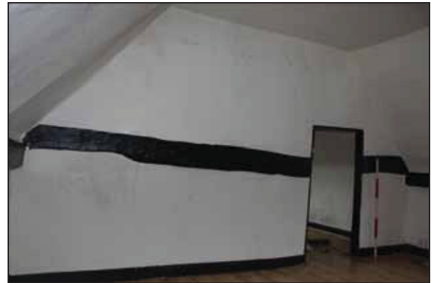
Marks within the paintwork possibly for original hinges, FF03, taken from the north-east
