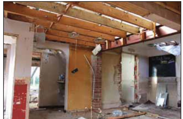
Original timber at the bay division acting as door jamb, south-east elevation, taken from the east
