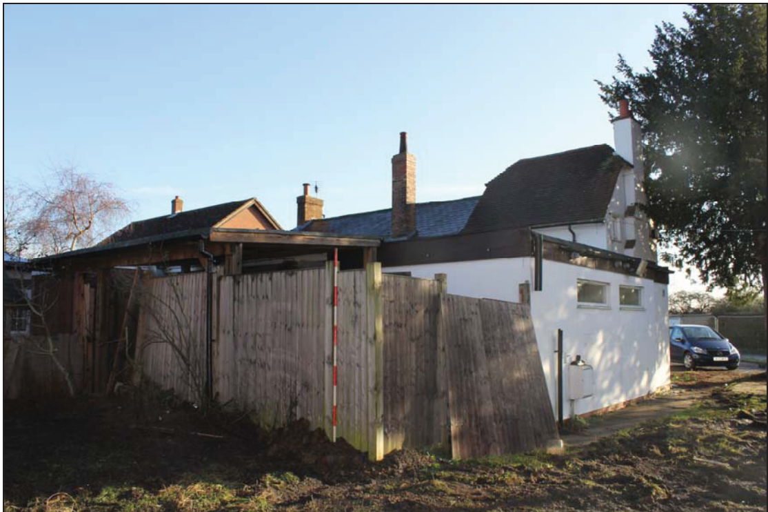
Plate 2 Rear of the Black Horse, taken from the west (DP 7)
