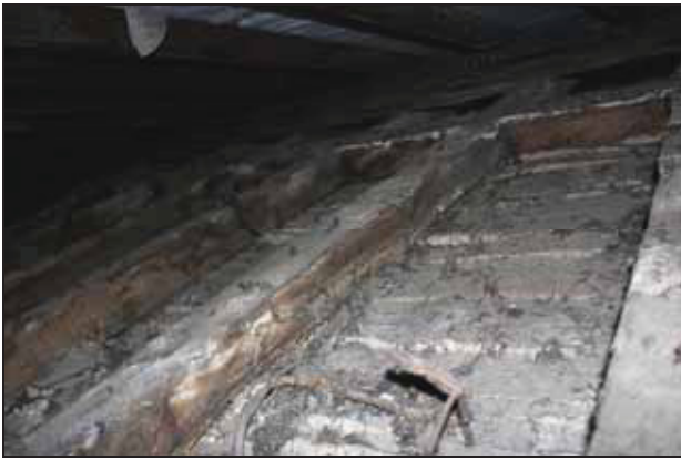
Original rafter feet preserved within pent-roofed extension seen from FF05, taken from the north-east
