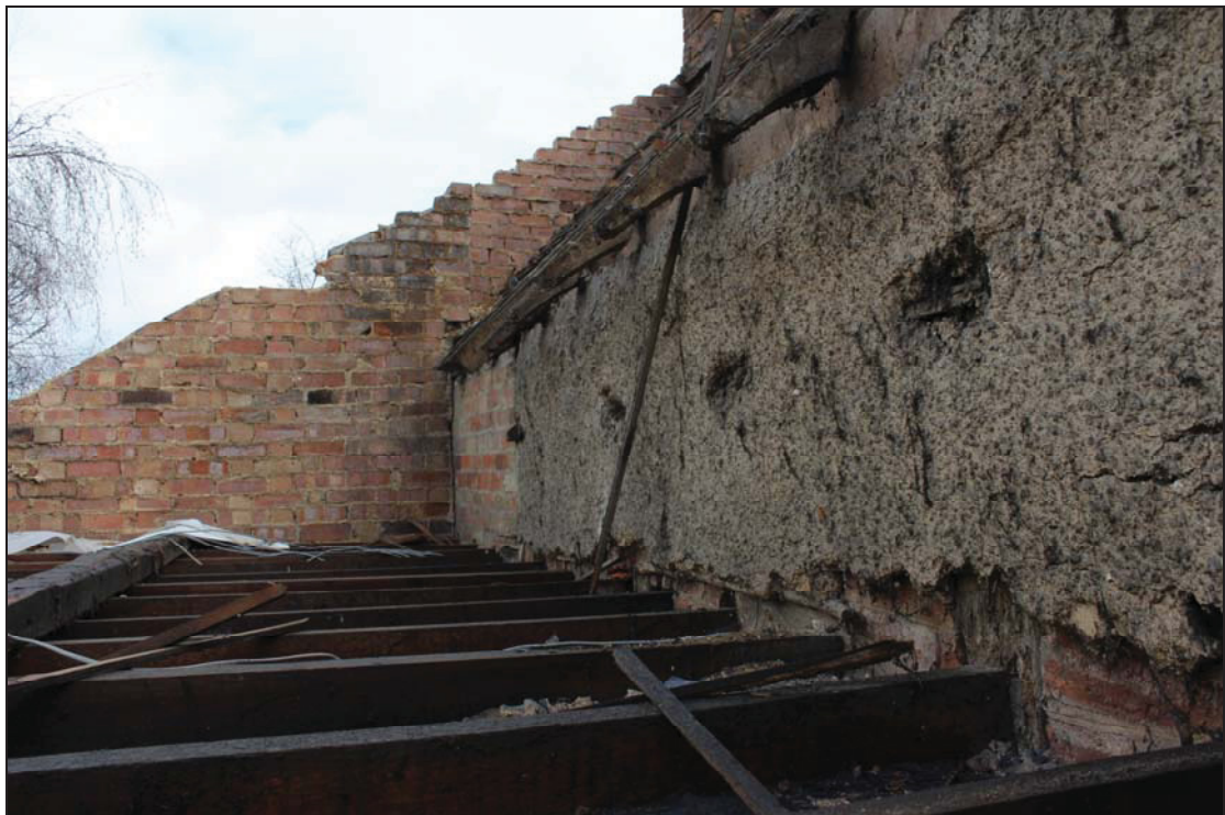
Plate 10 Sections of external render to north-west elevation, south-west (DP 81)
