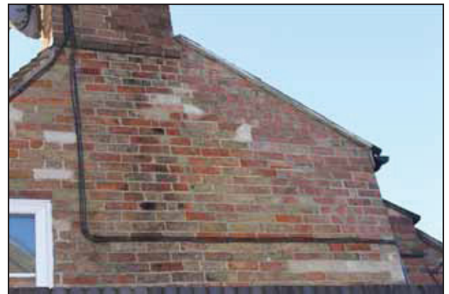
Evidence of the western roof pitch being raised, north-east elevation, taken from the north-east
