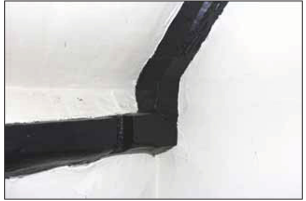
Tie-beam cut through to accommodate early 20 th century extension, FF01, taken from the north
