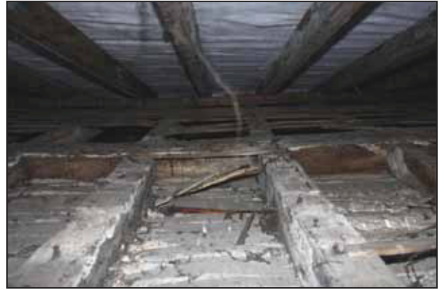
Common-rafters rising above and below a robust purlin seen from FF05, taken from the north-west
