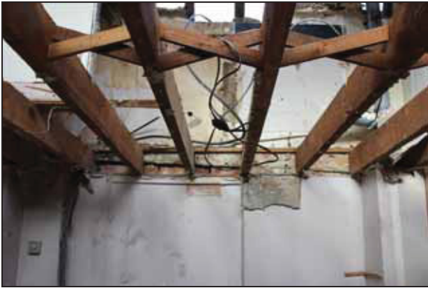
Modern joisting keyed into original mid-rail, GF02, taken from the south-east
