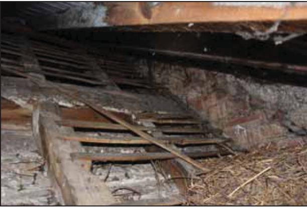
Surviving external batons once carrying peg-tiles at the junction with pent-roof seen from FF05, taken from the north-west
