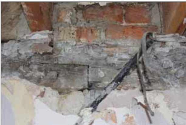
Timber-framing infilled with brick at the bay division, FF01, taken from the south-east
