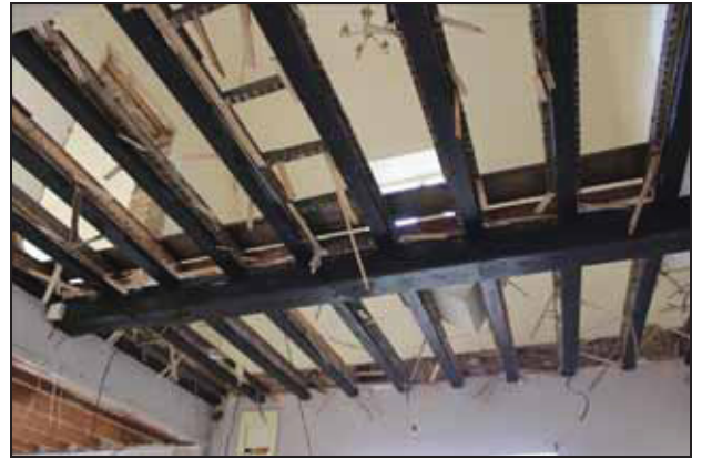
Floor joisting to south bay, GF02, taken from the north-west
