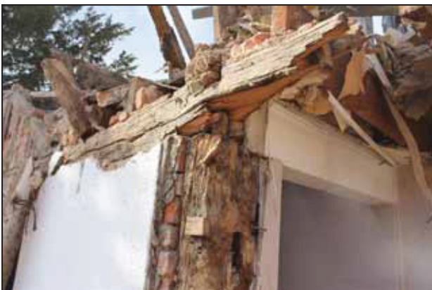
Principal-post morticed to the mid-rail, taken from the east
