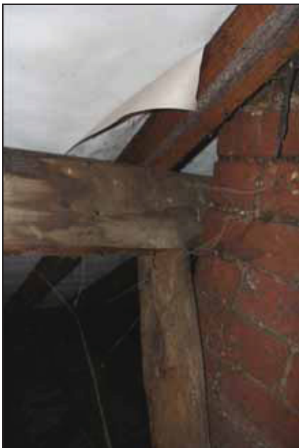
Common-rafters rising above and below a robust purlin seen from FF05, taken from the north-west
