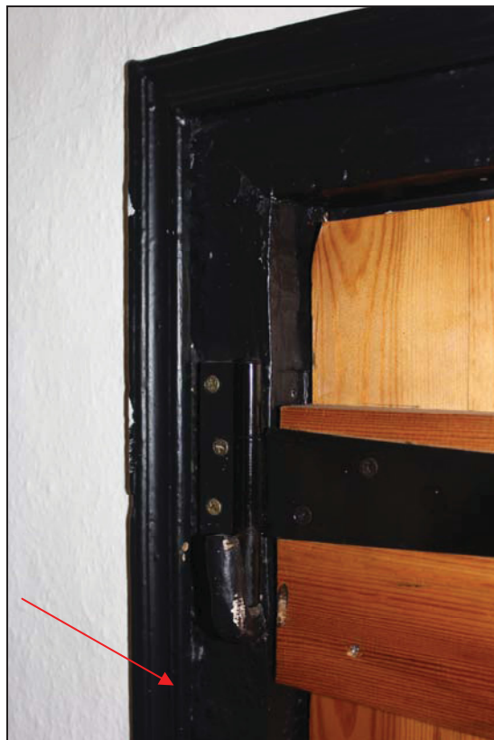
Plate 16 Surviving pintel to door frame, FF02, taken from the north (DP 42)
