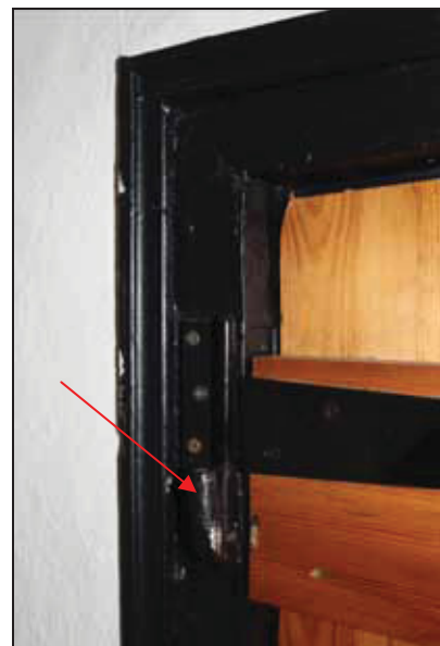
Surviving pintel to door frame, FF02, taken from the north
