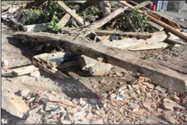
Purlin retaining mortices for common-rafters
