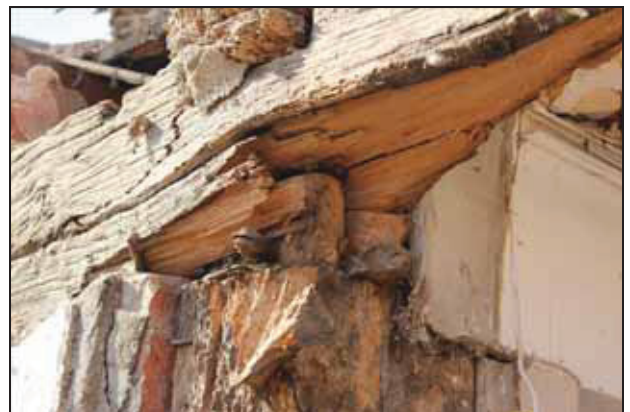
Principal-post morticed to the mid-rail, taken from the east
