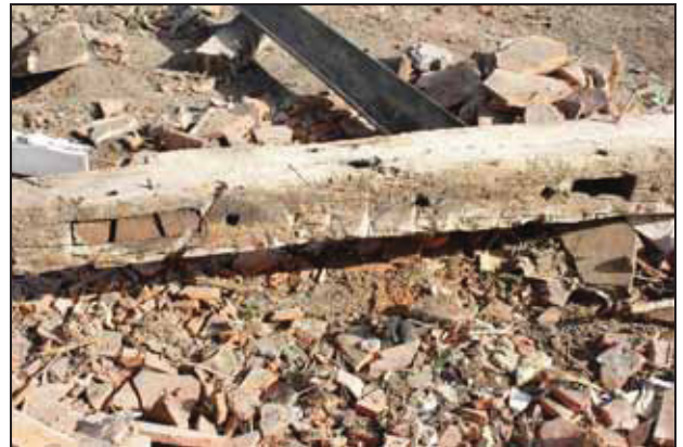
Mortices interspersed with stave holes for wattle and daub to mid-rail soffit
