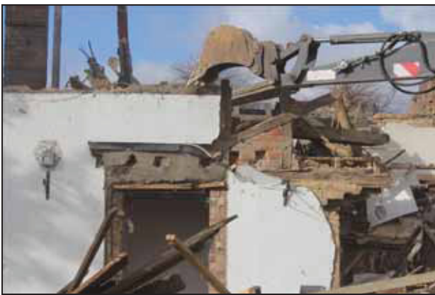
Removal of render to expose upper timber-framed sections, taken from the south-east
