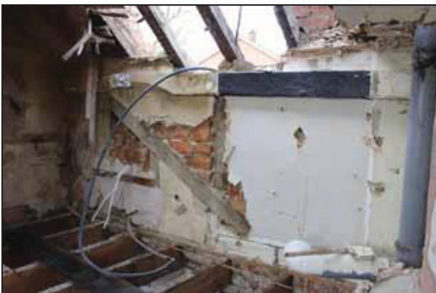
Primary braced studwork with brick infill to north-west elevation, FF01, taken from the north-east
