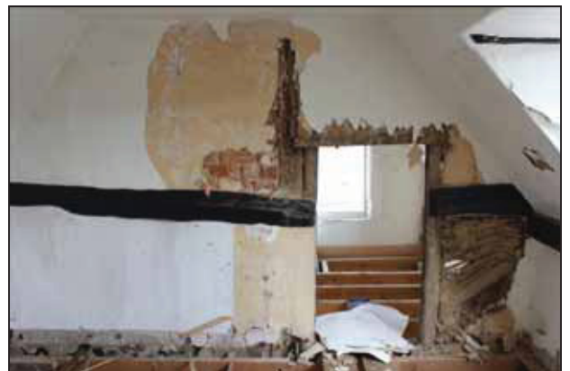
North gable preserving original timber-framing infilled with wattle and daub below the tie-beam, FF02, taken from the south
