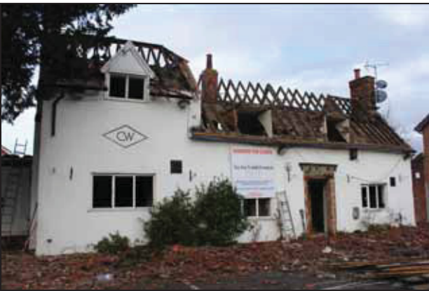
Surviving external batons once carrying peg-tiles at the junction with pent-roof seen from FF05, taken from the north-west
