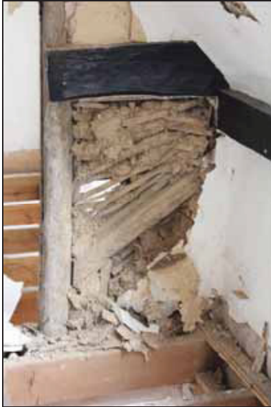
Wattle and daub infill around a brace, north gable, FF02, taken from the south-west
