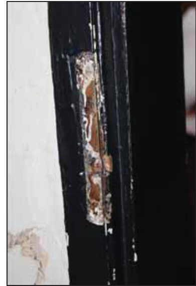
Marks within the paintwork possibly for original hinges, FF03, taken from the north-east
