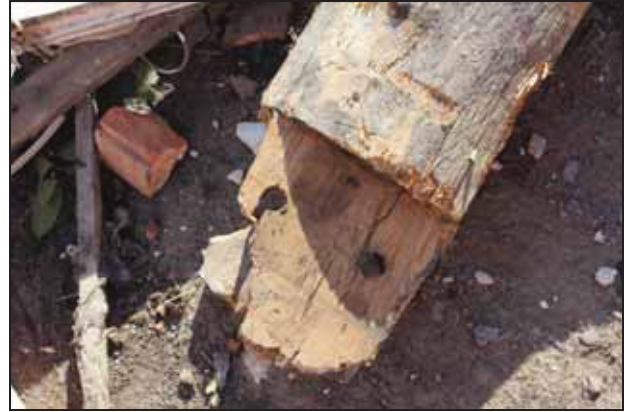
Double pegged mortice to purlin
