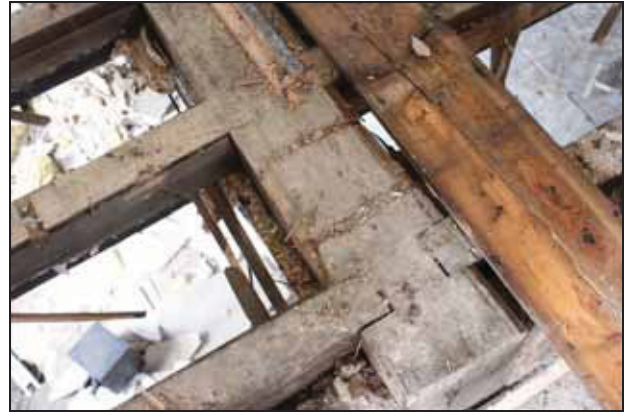
Impressions of studs and a brace, north gable, FF02, taken from the south
