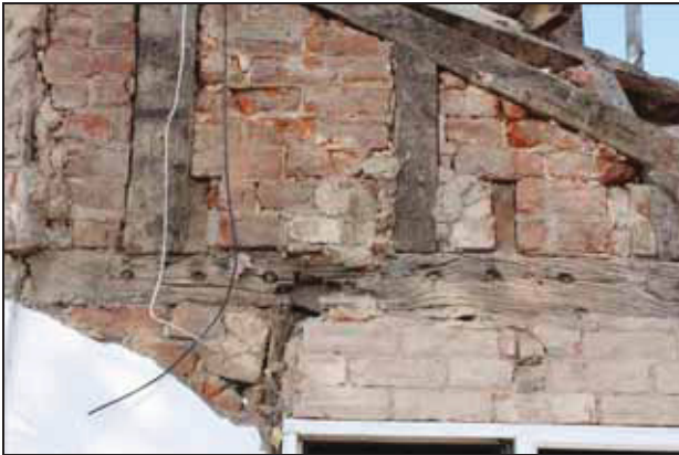
Upper timber-framed sections with pegging for a scarf joint in the mid-rail, taken from the south-east
