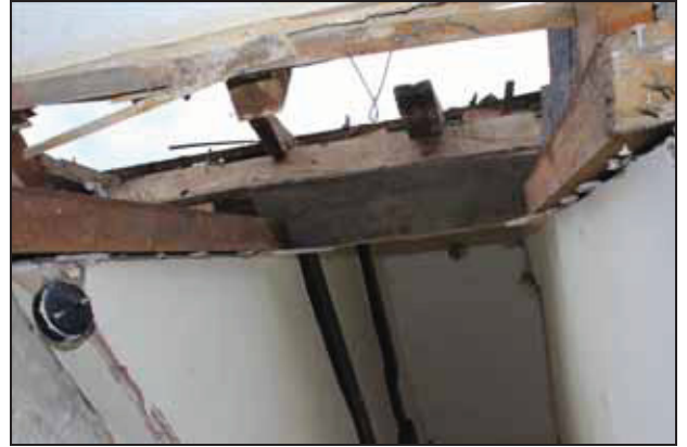
Original wall-plate extending along north-west elevation of historic core, GF04, taken from the north-west
