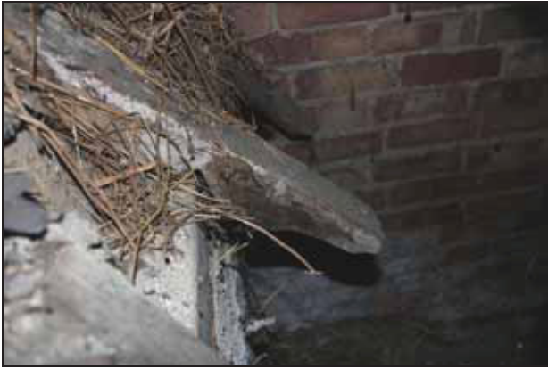
Original rafter feet preserved within pent-roofed extension seen from FF05, taken from the north-east
