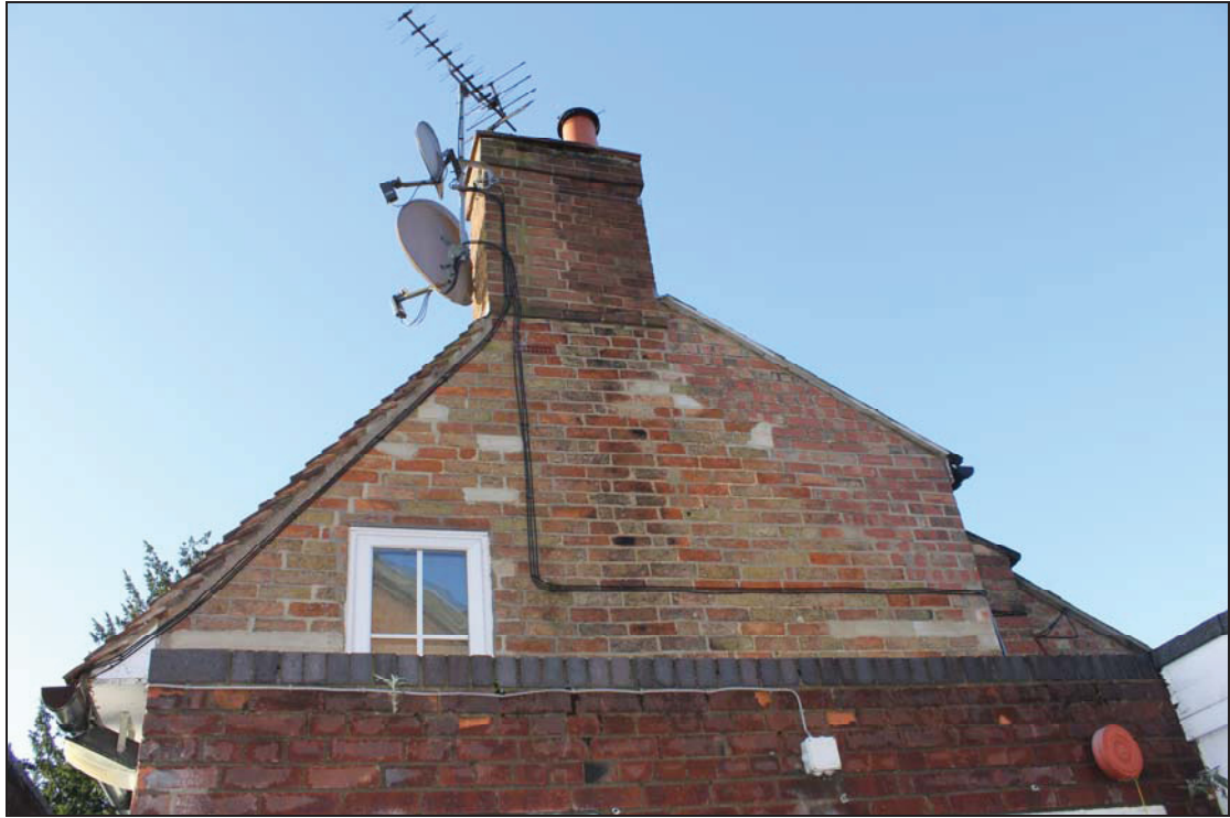
Plate 3 Upper sections of the north-east elevation, taken from the north-east (DP 11)
