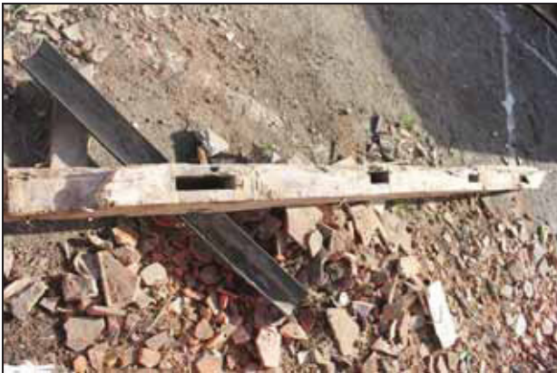
Mid-rail with empty mortices for studs to soffit
