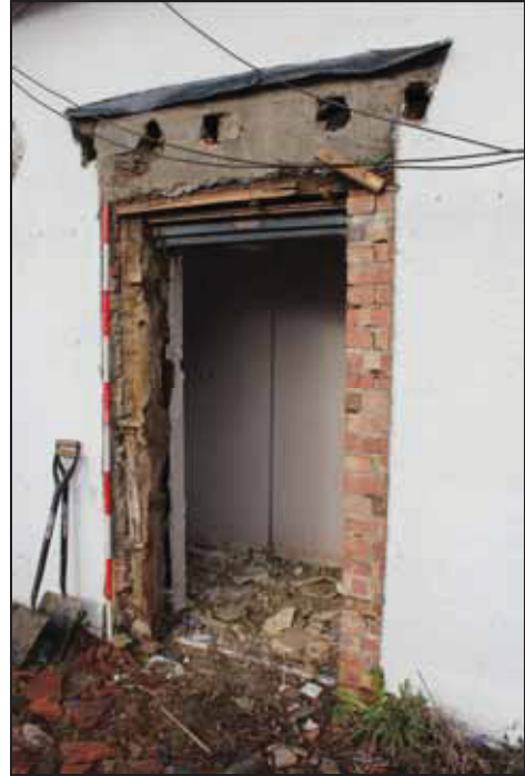
Original timber at the bay division acting as door jamb, south-east elevation, taken from the east
