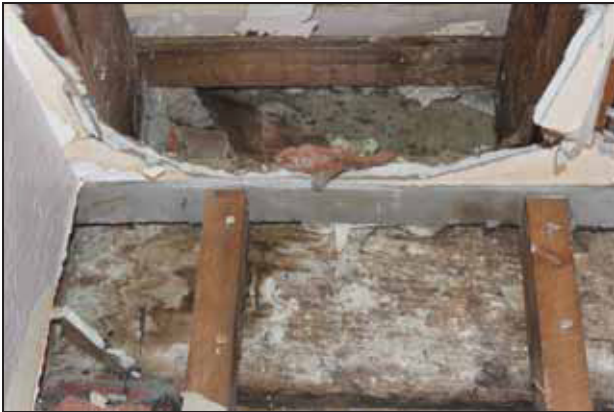
Downward brace extending to mid-rail above the main entrance, GF01, taken from the north-west
