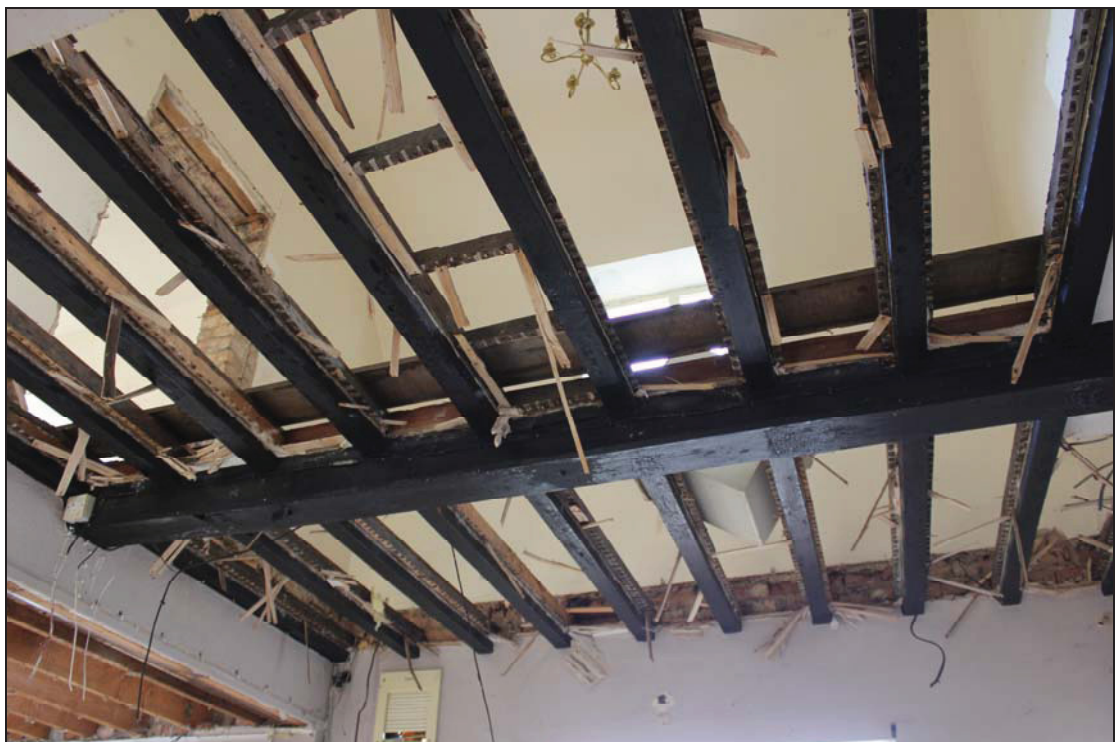
Plate 6 Floor joisting to south bay, GF02, taken from the north-west (DP 74)
