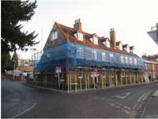
DP 1: Frontage of the former Black Lion Inn (looking NE)
