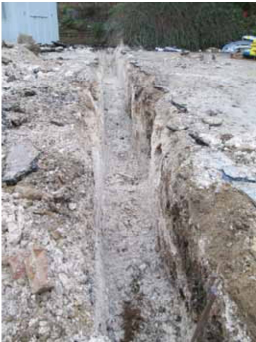
DP 5: Trench for new eastern boundary wall (looking NE)
