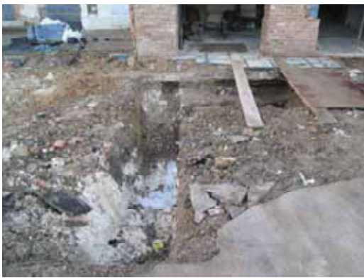
DP 3: Trench for the new building extension (looking SSW)
