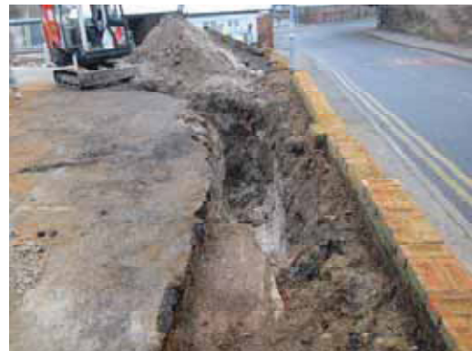
DP 10: Trench for new western boundary wall (N) (looking SW)
