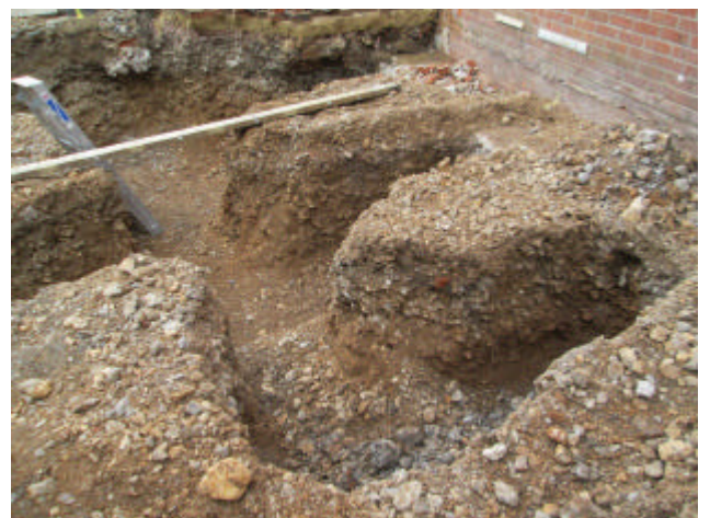
DP 12. North-western foundation trench. Looking west.
