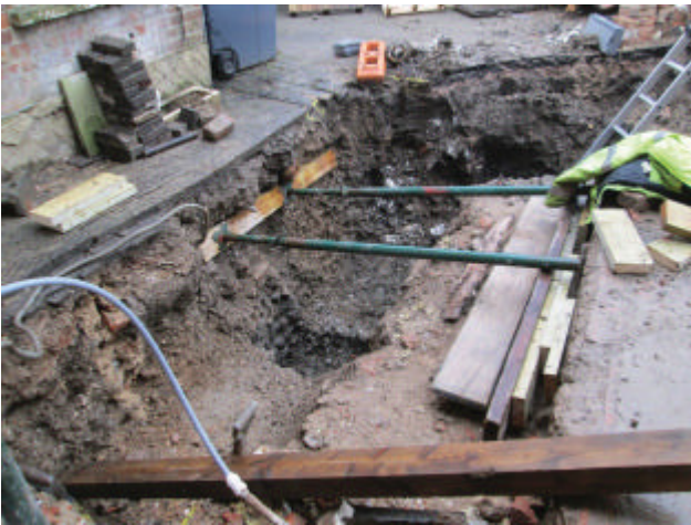
DP 3. South-west foundation trench. Looking west.
