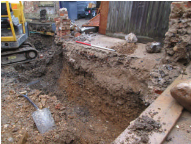
DP 9. Western foundation trench. Looking south.
