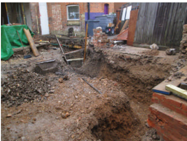
DP 11. Western foundation trench. Looking south.
