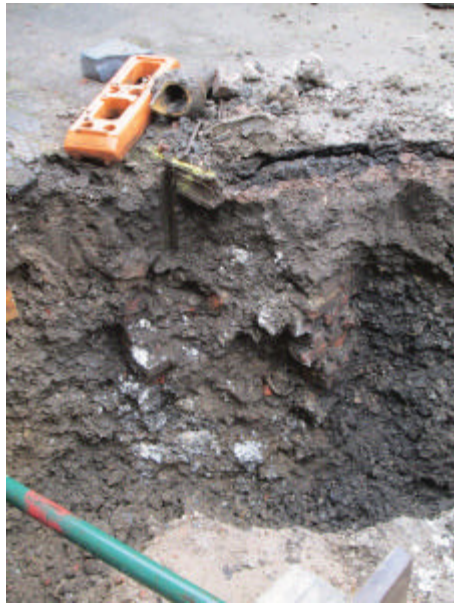
DP 7. Soakway F1024. Looking south-west.
