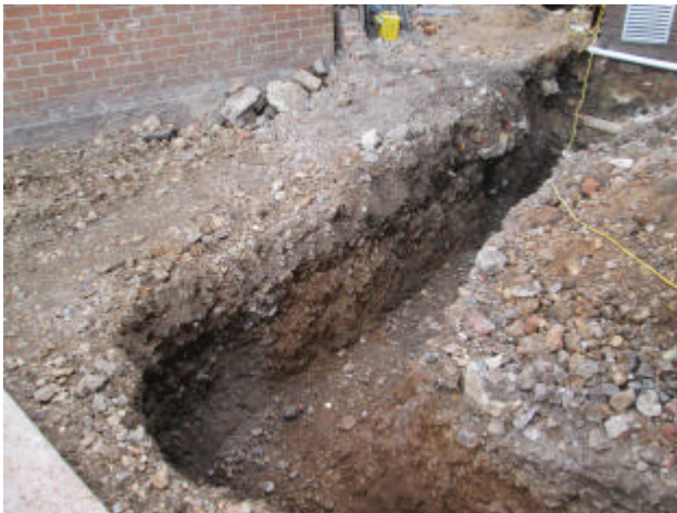
DP 15. Central foundation trench. Looking north..
