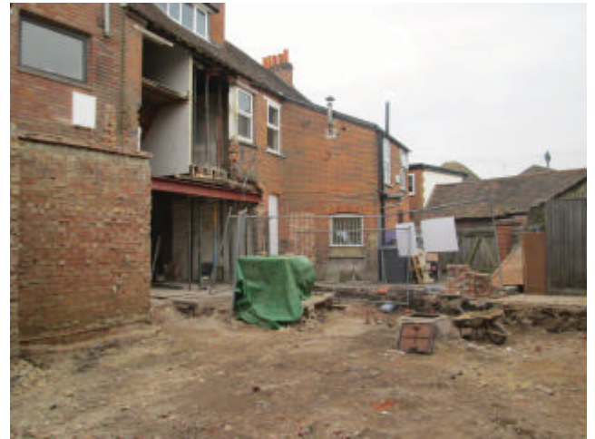
DP 2. Rear of the site. Looking south.
