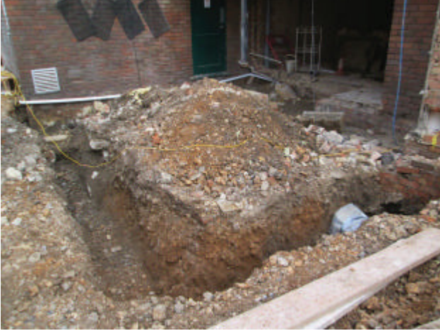
DP 13. Central foundation trench. Looking north-east.
