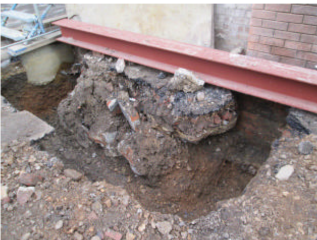
DP 17. Northern foundation trench. Looking north-east.
