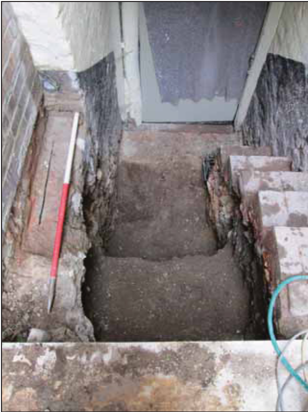
1 View of works, facing north-northeast
