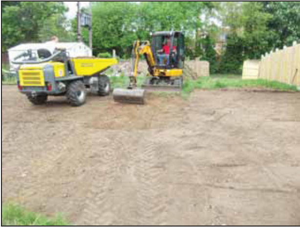
1 General shot of site at commencement of strip
