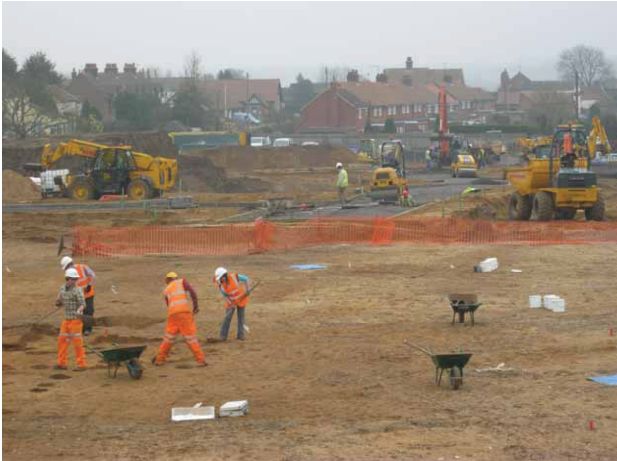
Plate 2: Site record shot (during excavation/ development (looking S)
