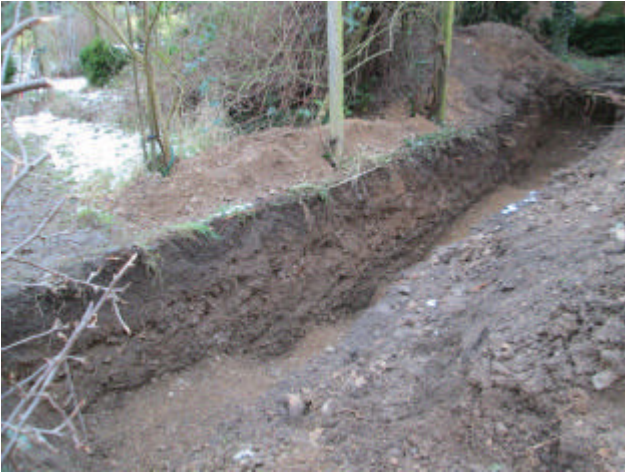
DP 3. Trench 1. Looking north-west.
