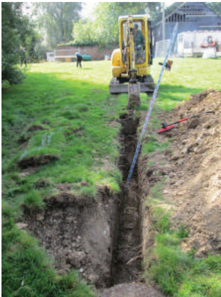
DP 3. Drainage trench. Looking south.
