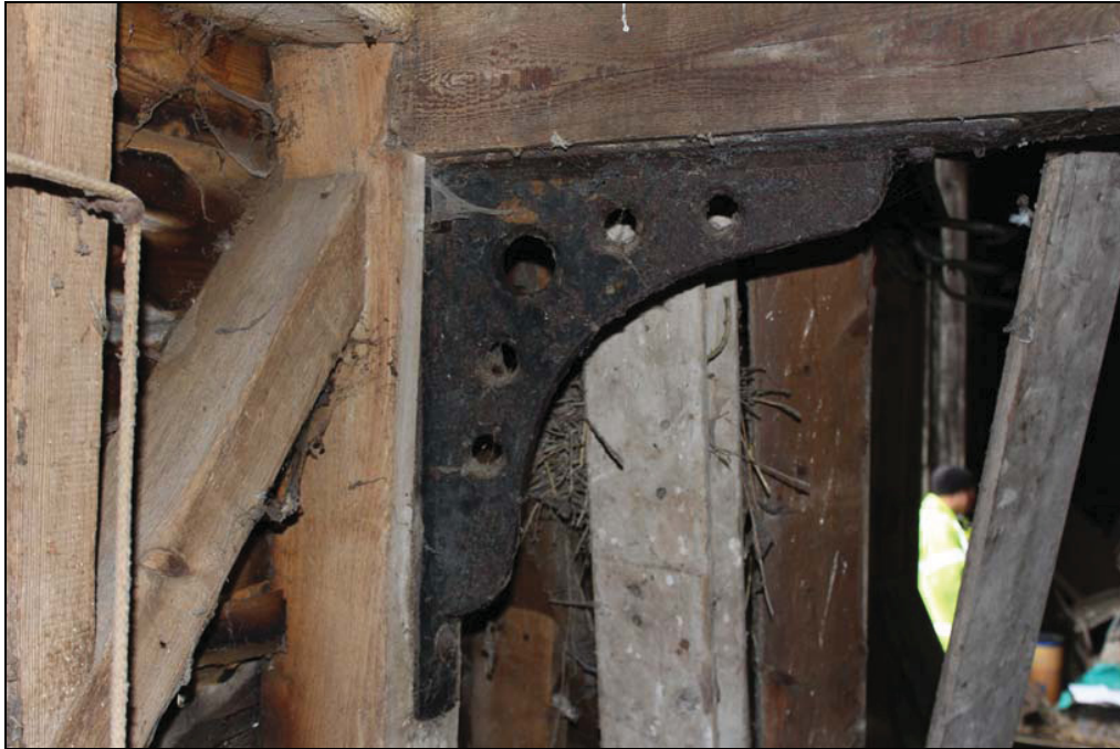
Plate 7 Decorative iron brace to tie-beam, Bay 4, taken from the south (DP 10)
