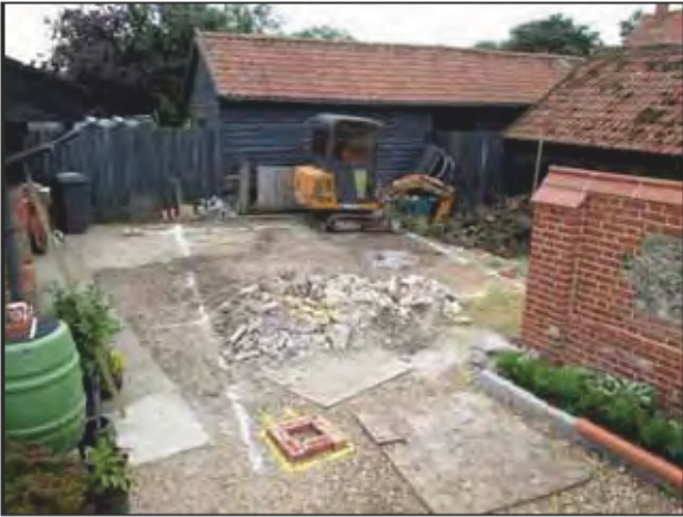
1 General site shot before commencement of works
