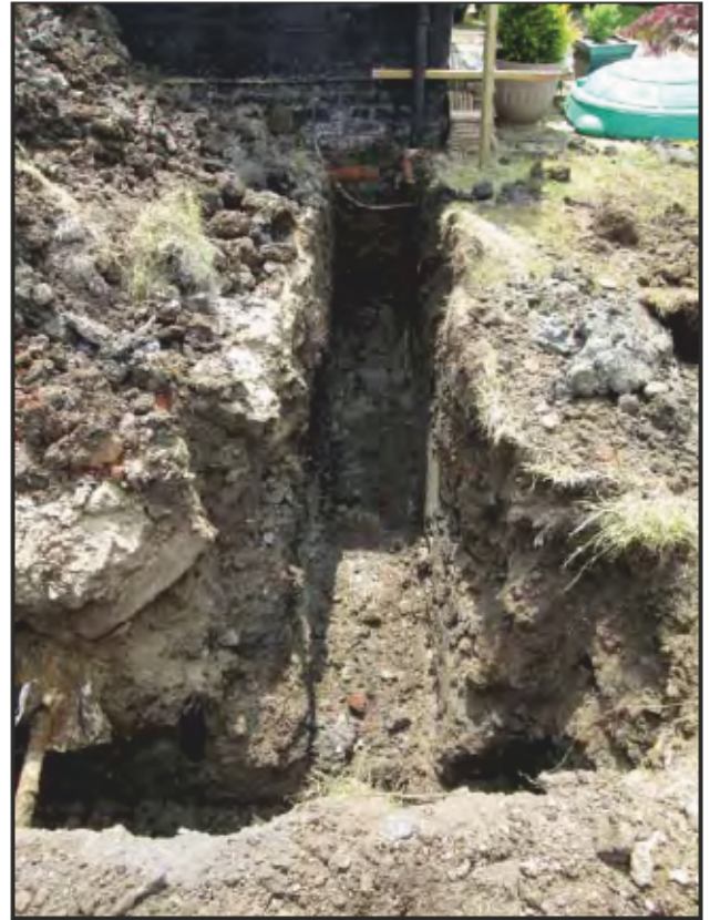
2 View of footings
