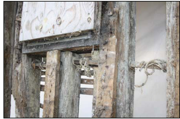
Wattle and daub staves in situ west elevation of cross-wing, taken from the west
