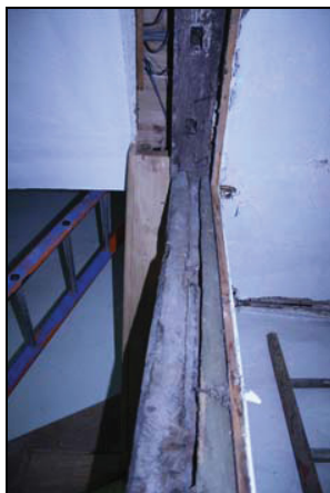
Redundant mortices for a window located along the mid-rail at junction between the cross-wing and the central hall range, taken from the north-west
