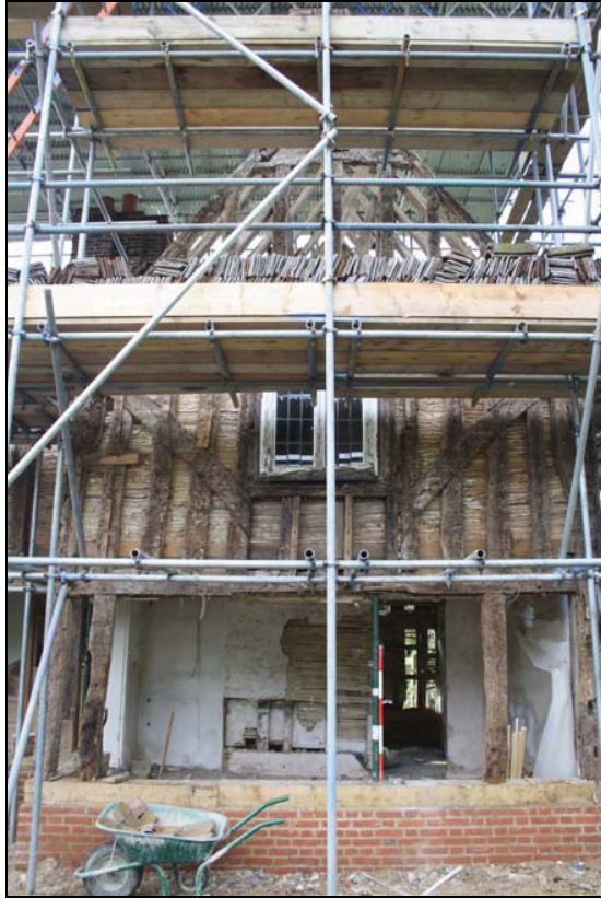
Plate 3 Cross-wing, timber-frame fully exposed, north elevation, taken from the north-east (DP 60)
