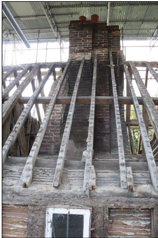
Plate 10 Chimney stack clasped by rafters, taken from the north-west (DP 85)
