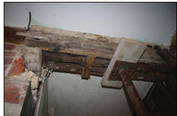
Redundant mortices for studwork located along the mid-rail at junction between the cross-wing and the central hall range, taken from the east
