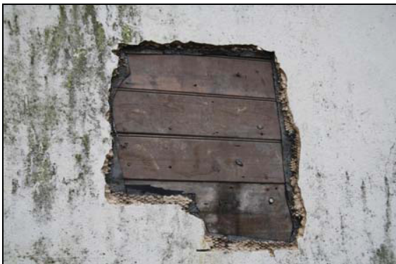
Match-lined boarding beneath the render, north elevation, taken from the north-east
