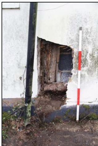
Crude weatherboarding beneath the render, west elevation, taken from the north-west
