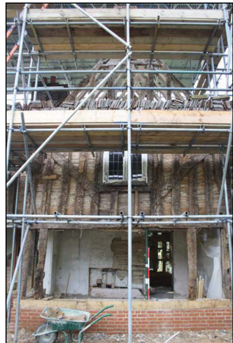
Downward brace cogged over studwork, west elevation of cross-wing, taken from the north-west
