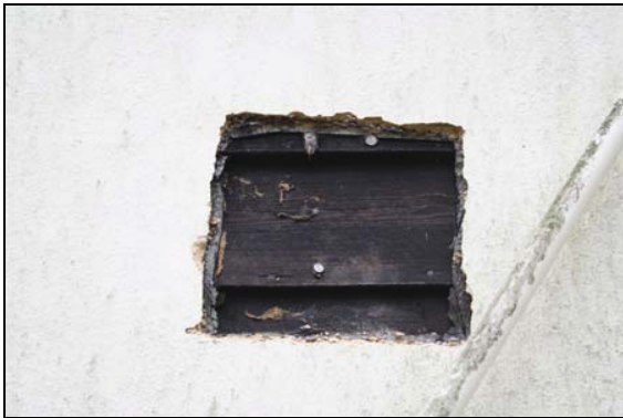
Render and weatherboarding removed exposing timber frame below, south elevation, taken from the south-west
