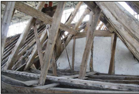
Windbraces, part of cross-wing roof construction, taken from the west
