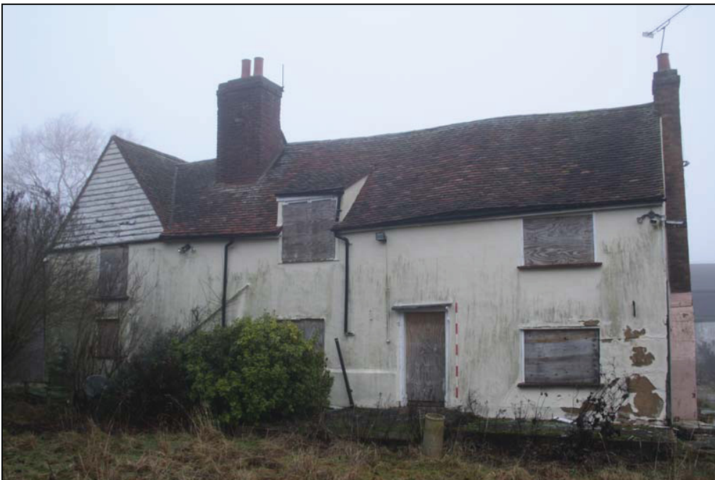
Plate 2 The Pond House, southern elevation, taken from the south-east (DP 1)
