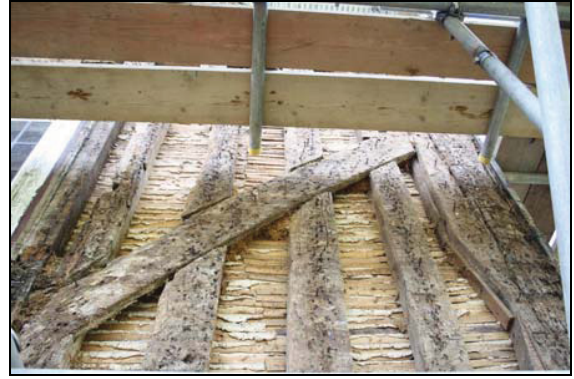
Brace and jowled corner-post, upper floor of cross-wing, timber-frame fully exposed, north elevation, taken from the north-east
