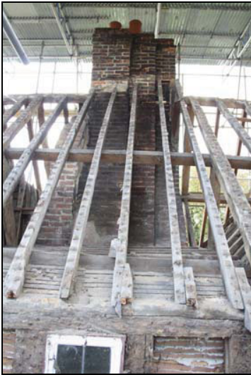
Chimney stack clasped by rafters, taken from the north-west
