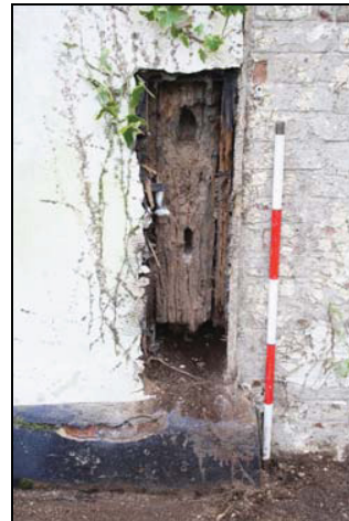
Exposure of the north-east corner-post, taken from the north-east
