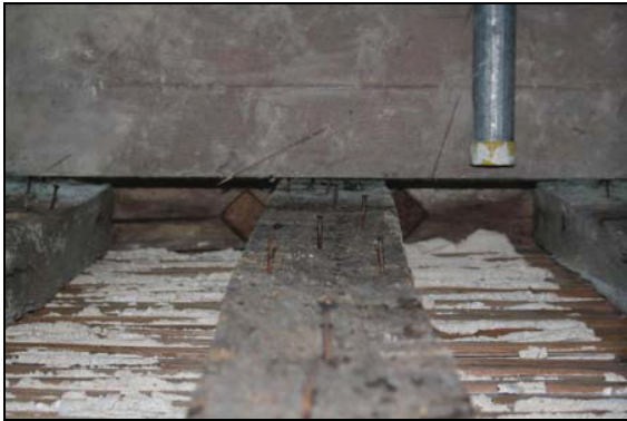
Diamond mullions located on the underside of the wall-plate, west elevation of cross-wing, taken from the north-west
