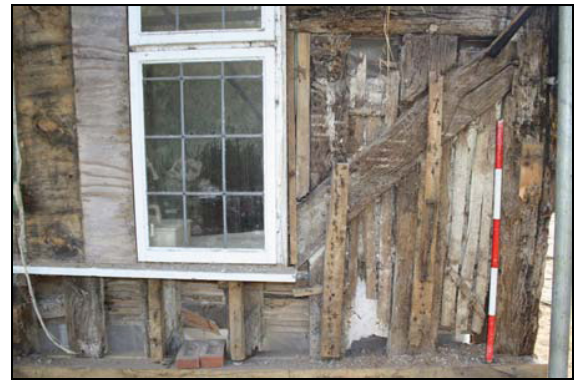
Wattle and daub staves in situ west elevation of cross-wing, taken from the west
