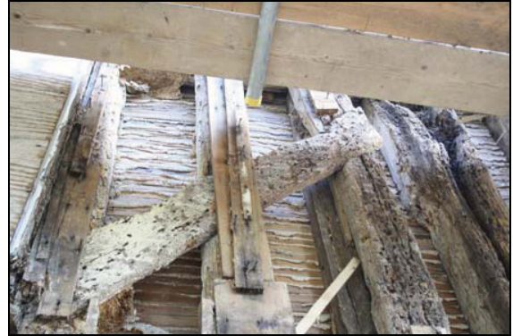
Brace, cogged over studs at first floor level, cross-wing, south elevation, taken from the south-west
