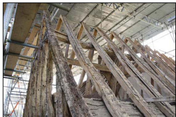
Even pattern of stave holes to the studwork, northern gable of the cross-wing, taken from the north
