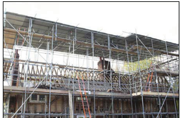
Brace and jowled corner-post, upper floor of cross-wing, timber-frame fully exposed, north elevation, taken from the north-east
