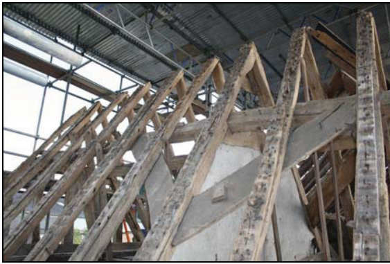
Windbraces, part of cross-wing roof construction, taken from the west
