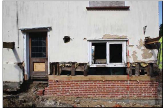
New dwarf-wall with exposed studs, south elevation, taken from the south-west
