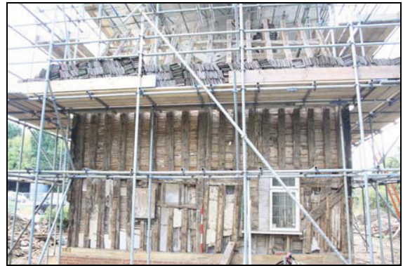
Brace, cogged over studs at first floor level, cross-wing, south elevation, taken from the south-west
