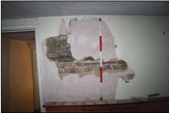
Plasterwork partially removed above the fireplace revealing a large timber bressummer, Room 1, taken from the south-east
