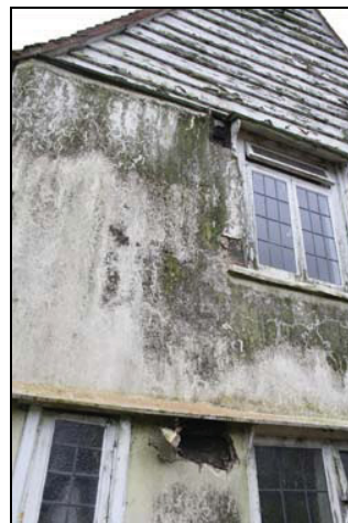
Two areas of render removed with weatherboarding beneath, cross-wing, north elevation, taken from the east
