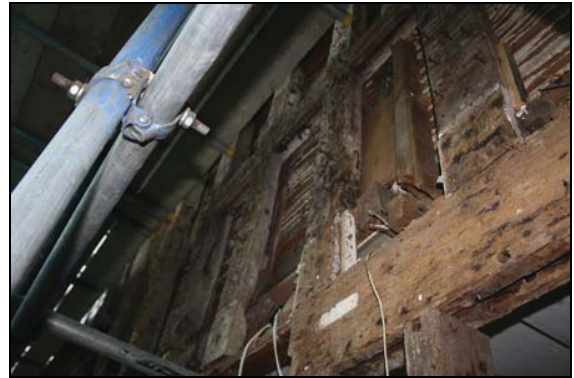
Wattle groove and stave holes to the studs and mid-rail, central hall range, taken from the north
