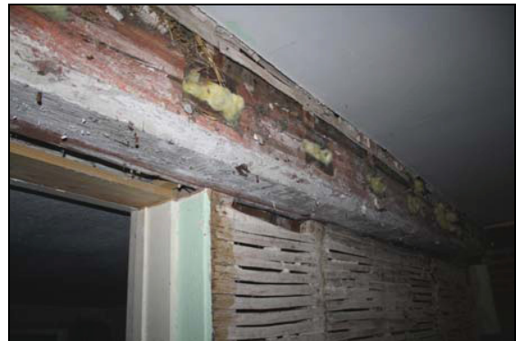
Central joist between Rooms 3 and 4 covered in red pigment with redundant mortices for common-joists, Room 4, taken from the west
