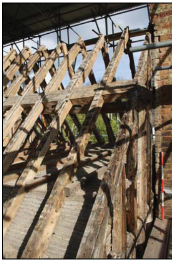
Common-rafters above and below robust purlins, roof above the kitchen range, north pitch taken from the north-east
