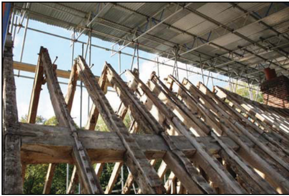
Common-rafters above and below robust purlins, roof above the kitchen range, north pitch taken from the north-east
