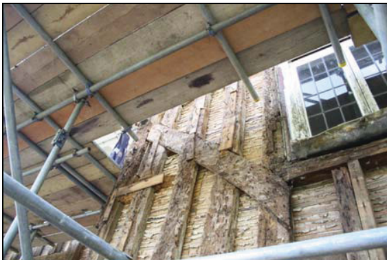
Brace and jowled corner-post, upper floor of cross-wing, timber-frame fully exposed, north elevation, taken from the north-east
