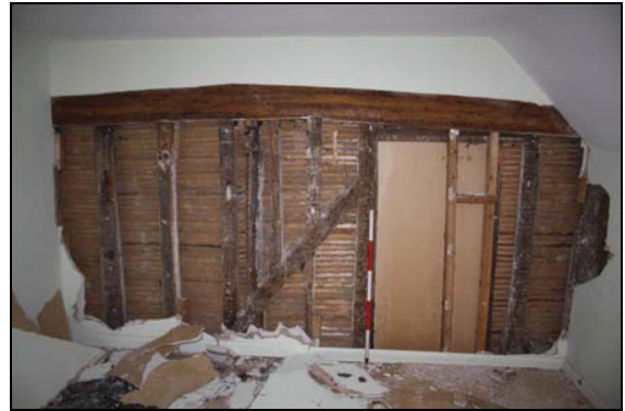
Modern wall coverings removed with studwork beneath, Room 7, taken from the north-west
