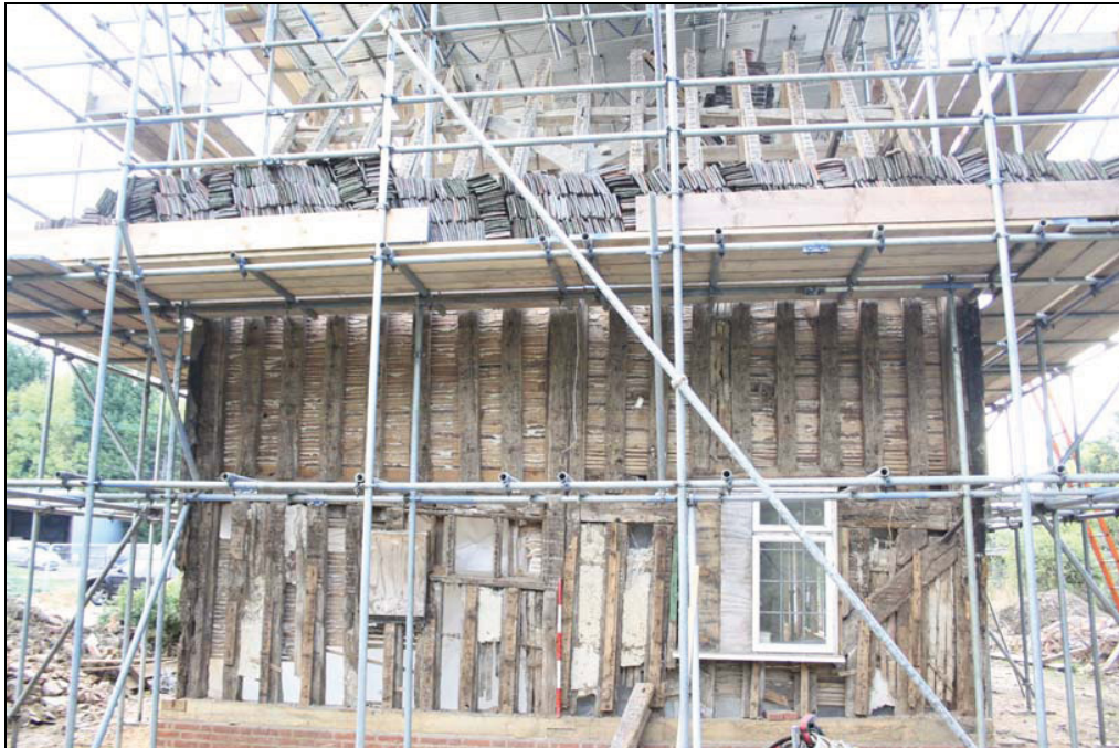
Plate 4 West elevation, timber-frame fully exposed, taken from the north-west (DP 52)
