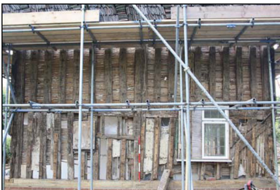
Brace, cogged over studs at first floor level, cross-wing, south elevation, taken from the south-west
