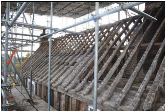
Chimney stack clasped by rafters, taken from the north-west
