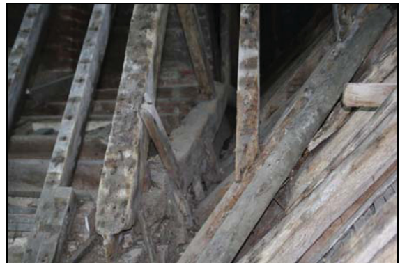
Junction between central hall range and the cross-wing, wane trusses either side of the chimney, taken from the north-east
