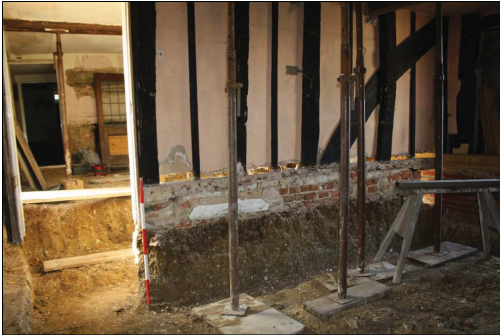
Plate 13 Lowering of floor levels, Rooms 1 & 2, taken from the south-east (DP 32)
