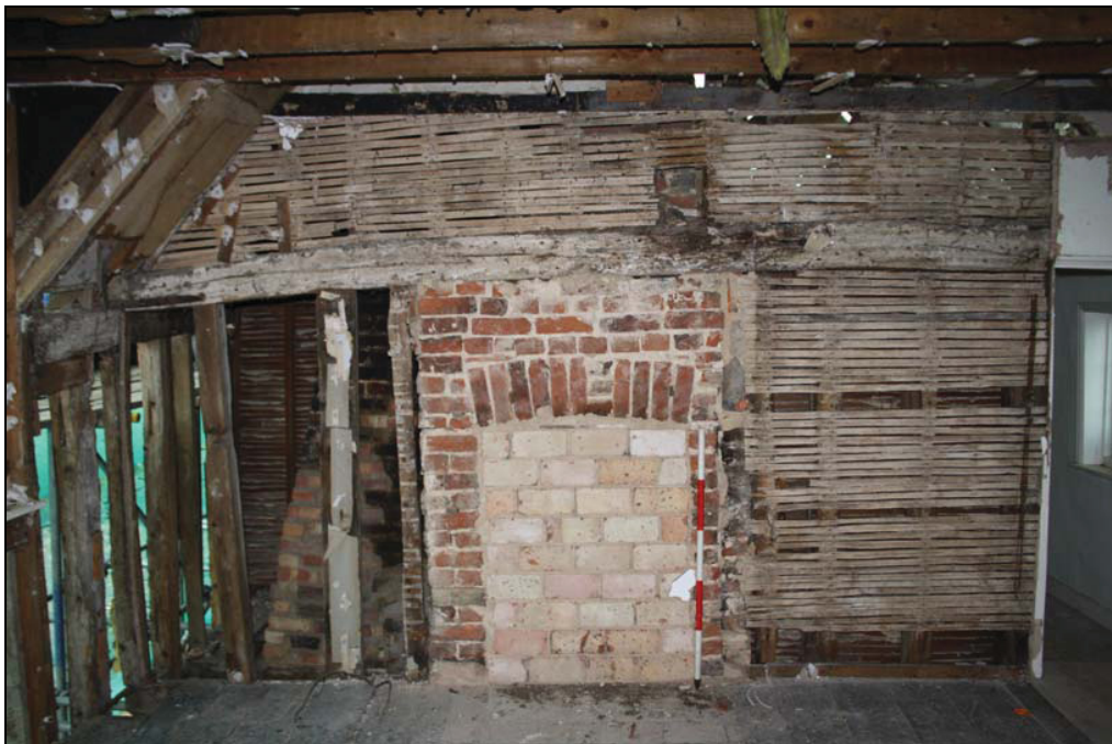
Plate 12 Blocked fireplace, Room 7, first floor, taken from the south-east (DP 88)
