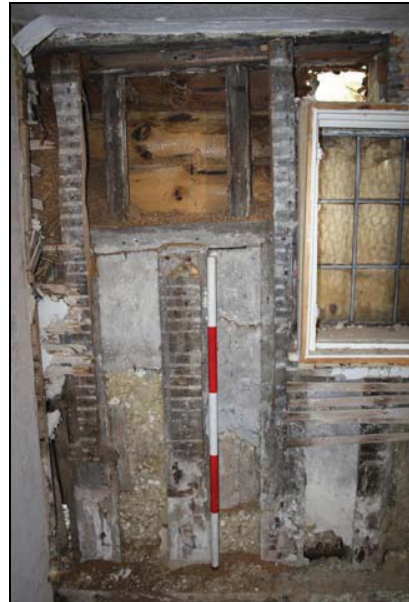
New dwarf-wall with exposed studs, south elevation, taken from the south-west
