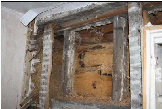
Early 17 th century window with ovolo moulded mullions and fillets, Room 3, taken from the east
