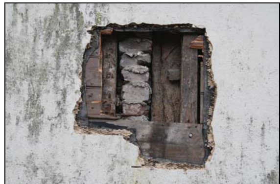
Render removed to reveal corner post in a poor condition, south-east corner of the building, taken from the east
