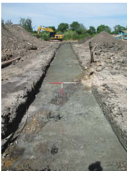
DP 17. Trench 5. Looking north-east.
