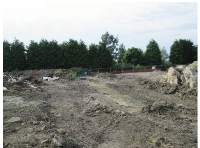
DP 12. North-east part of the site with Trench 4. Looking south-south-east.
