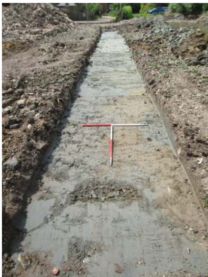
DP 5. Trench 2. Looking north-east.
