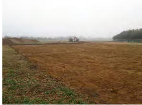
4: Topsoil stripping (NW site area), looking SE
