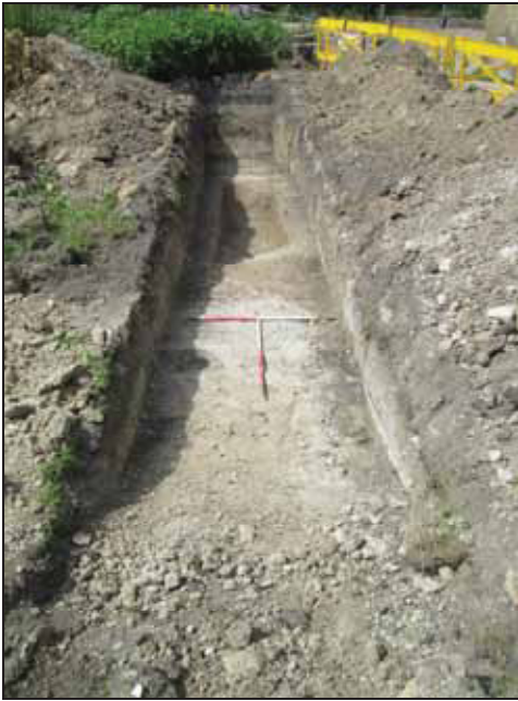
9 Trial trench 3, facing northwest
