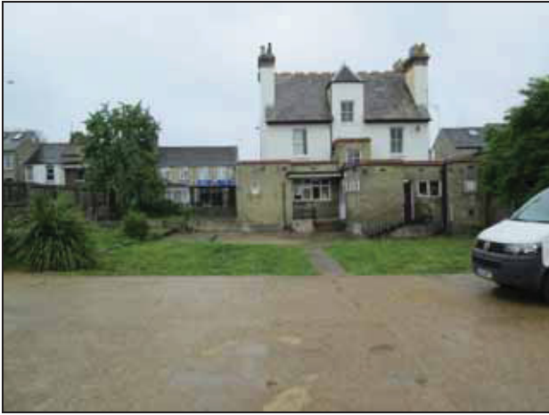
1 View across the site, facing northeast
