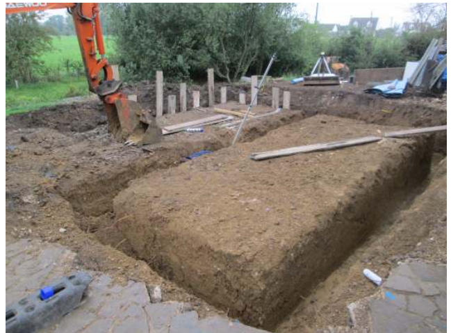
DP 2. Foundation trenches. Looking south-west.
