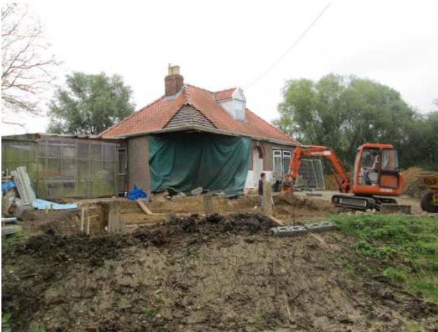
DP 1. The site of new garage. Looking north-east.
