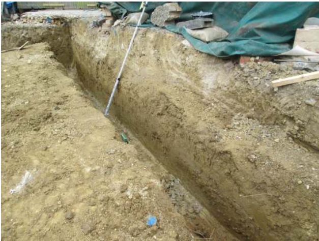
DP 3. North-east trench. Looking north-north-west.
