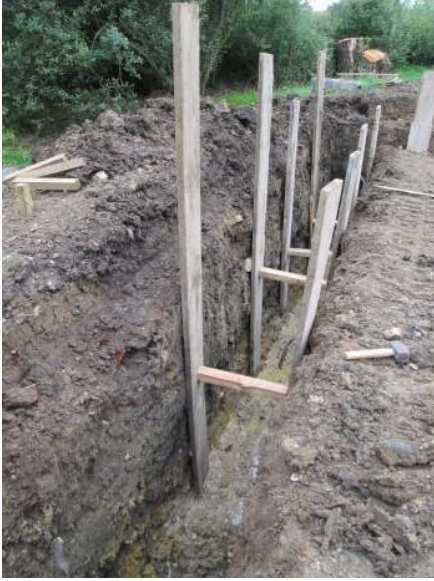
DP 7. South-west trench. Looking west-north-west.
