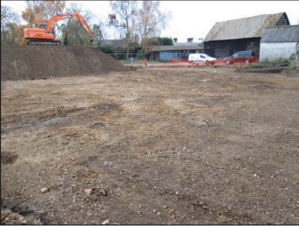
1 View facing north across the site
