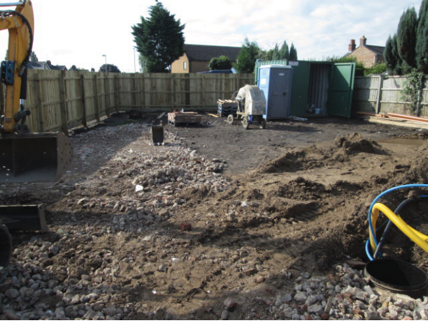
1 General shot of site before excavation
