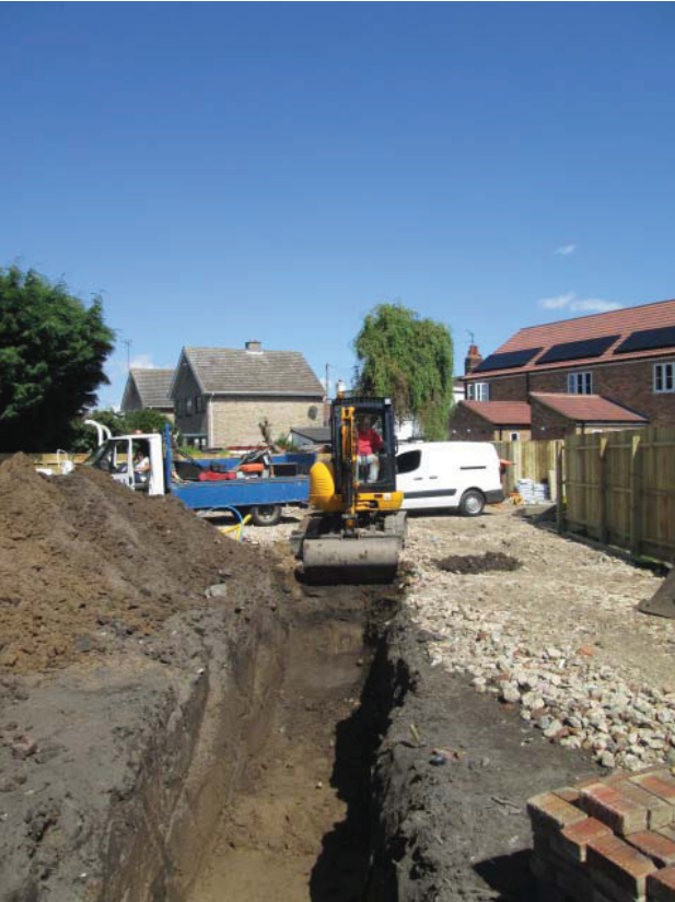
3 Trench being excavated
