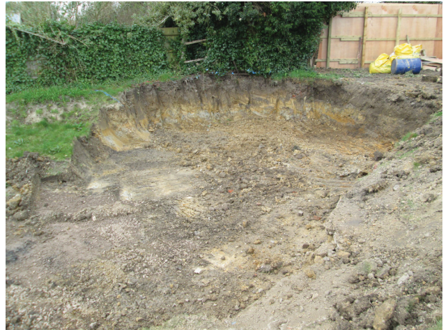
DP 2. North-west corner of the site. Looking north-north-west.
