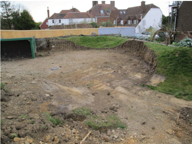
DP 3. South-east part of the site. Looking south-east.
