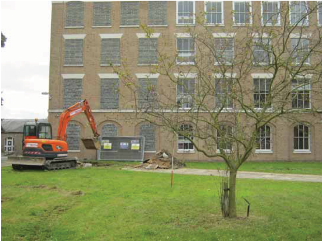
DP 1: General site shot (excavation commencing), looking SE
