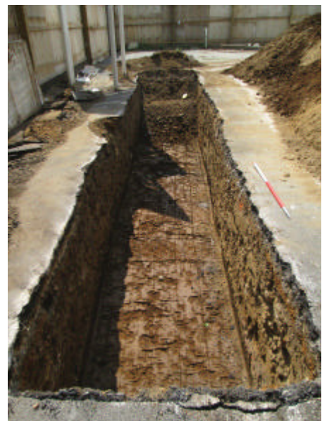
DP 10. Trench 3. Looking south-south-west.
