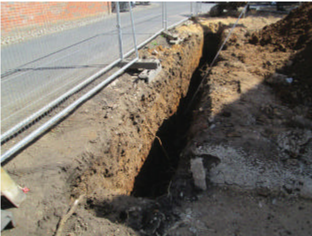
DP 9. North foundation trench. Looking north-east.
