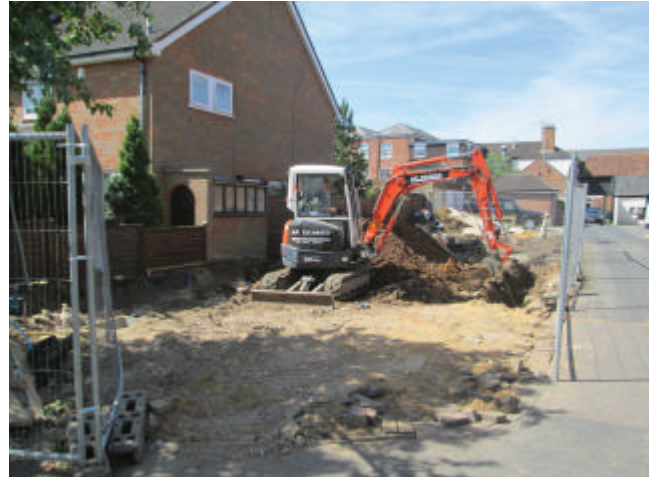
DP 2. The site. Looking south-west.
