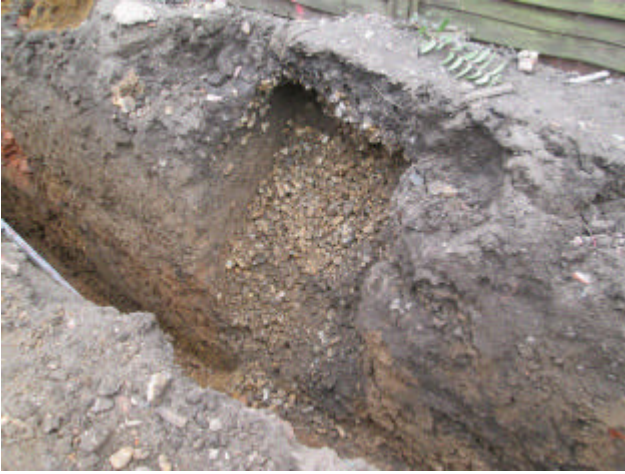
DP 7. South foundation trench. Modern soakway. Looking east-south-east.
