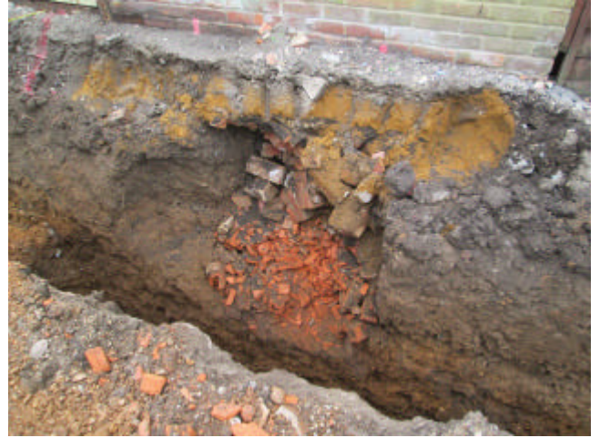
DP 8. South foundation trench. Modern soakway. Looking east-south-east.
