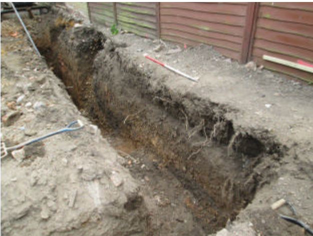
DP 5. South foundation trench. Looking east.
