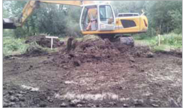
2 Topsoil and subsoil stripping looking south
