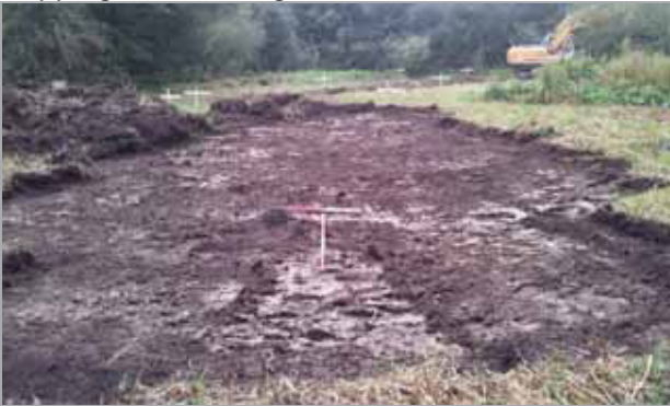
3 Complete stripping of the north area. Looking south
