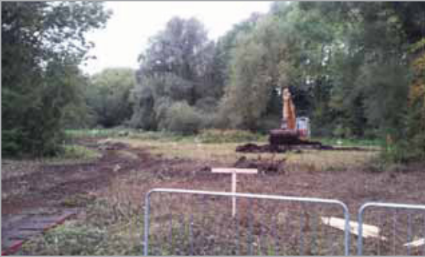
1 General site view looking south-west. Also topsoil stripping in the background
