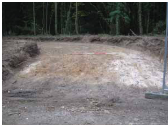
DP 19. Southern end of new access road (post-monitoring), looking NE
