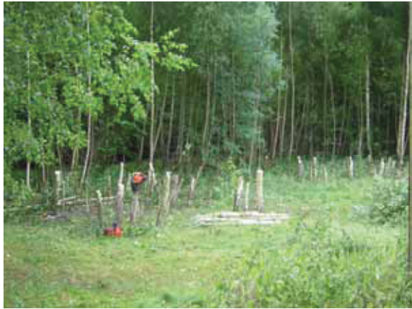
DP 3. Northern end of new access road (general shot; pre-monitoring), looking SE
