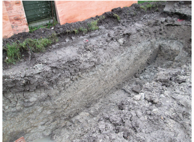
DP 2. West foundation trench during excavation. Looking north.
