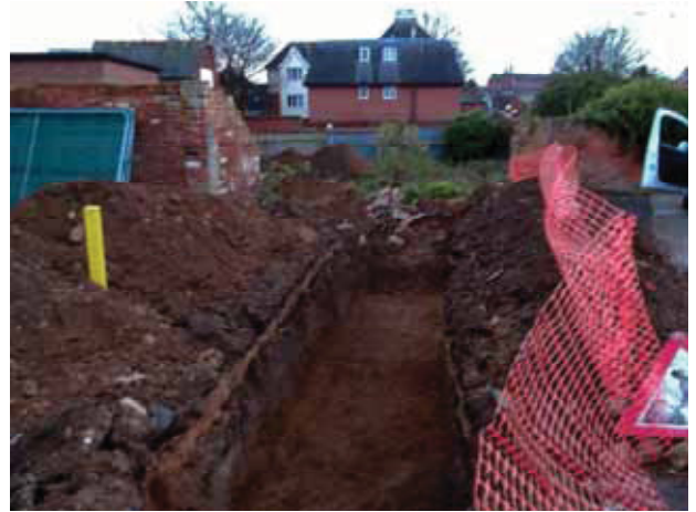
2 General view of the site. Looking north-west.
