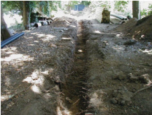
DP 9. Service trench. Looking north-north-east.
