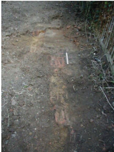
DP 7. Foundation Wall M2003. Looking north-north-east.
