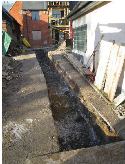
DP 54. Central part of service trench. Looking west-north-west.
