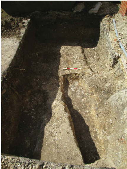
DP 3. New porch area excavation. Looking south-west.
