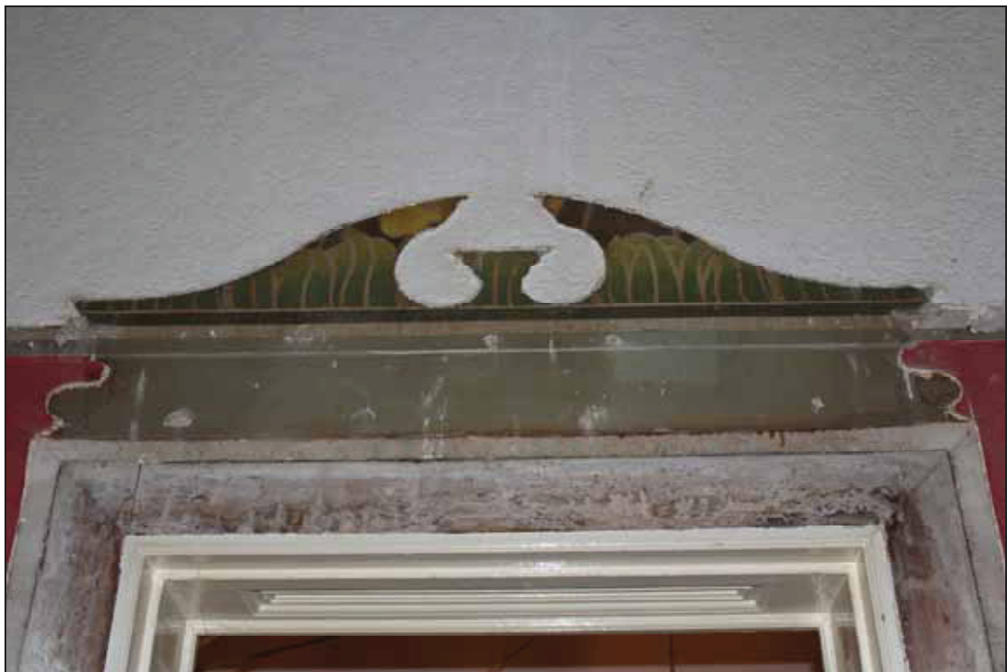
Plate 14 Wallpaper preserved beneath door case, GF05, taken from the north-east (DP 365)
