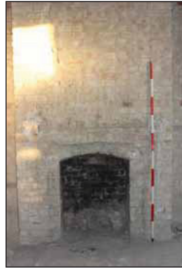
Chimney stack stripped back with removal of surround and grate, FF06, taken from the south-west
