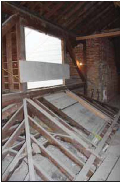
Hipped rafter arrangement surrounding central light well, SF09, taken from the south
