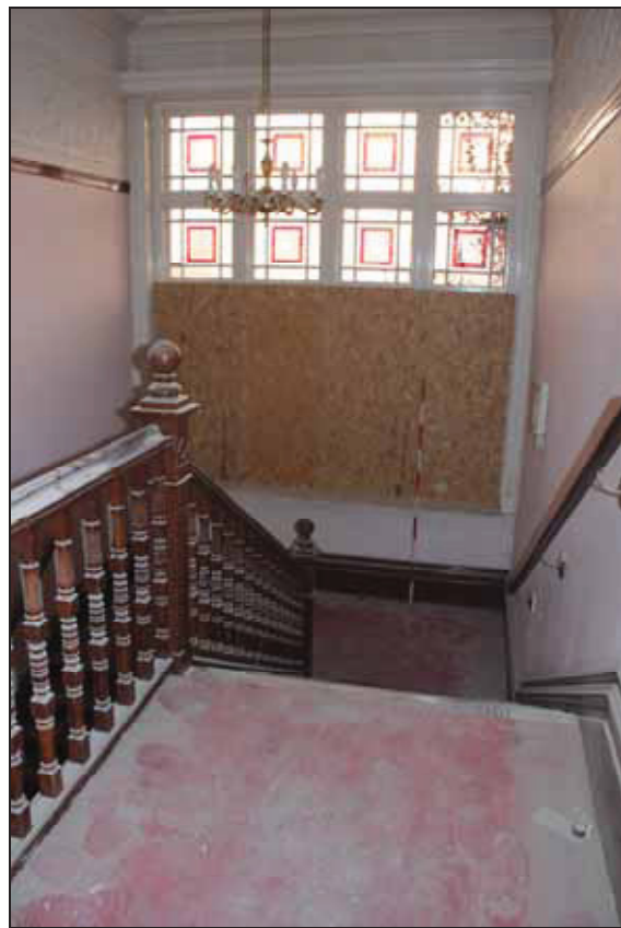
Plate 22 Staircase from first floor level, FF01, taken from the north (DP 233)
