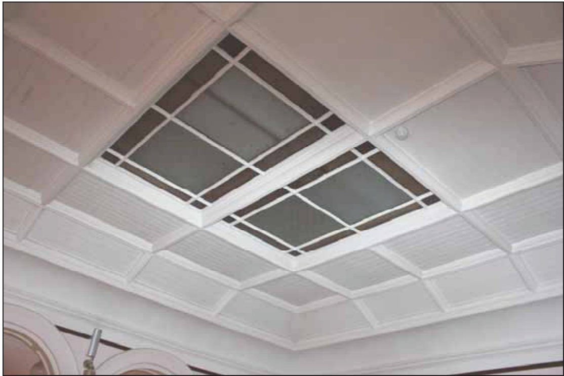
Plate 23 Ceiling above FF02, taken from the west (DP 350)
