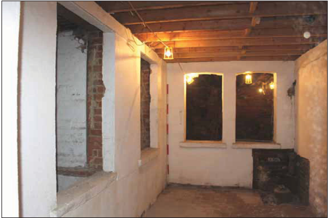
Plate 9 Original external space now boxed in and floored over, BF02, taken from the south (DP 112)
