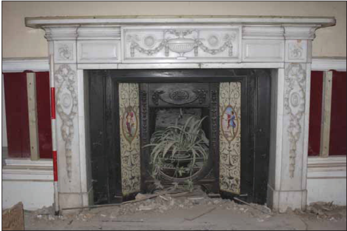
Plate 15 Fireplace with decorative reveals, GF06, taken from the south-west (DP 203)
