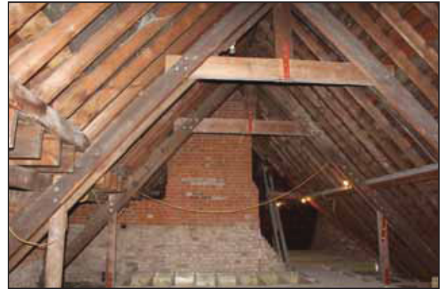
Timber hanger with Baltic mark, roof space above north gable, SF09, taken from the north
