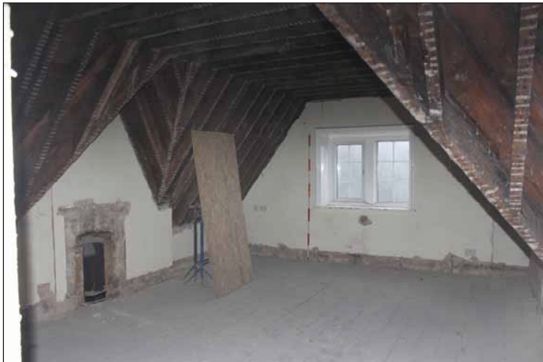
Plate 26 SF04, taken from the west (DP 308)
