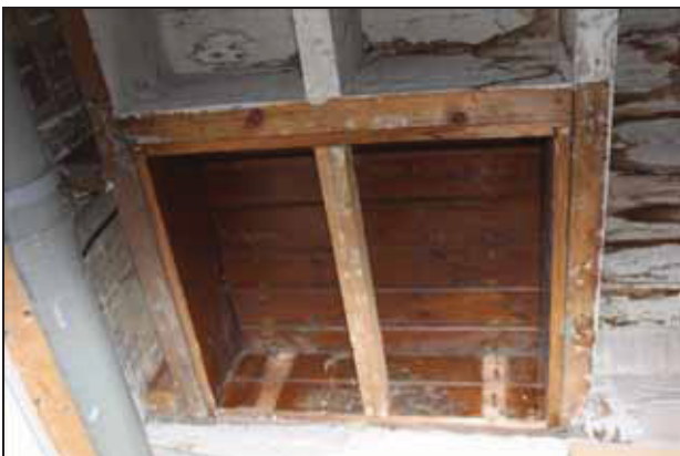
Original position of a staircase now infilled, GF06, north-east range, taken from the south-east
