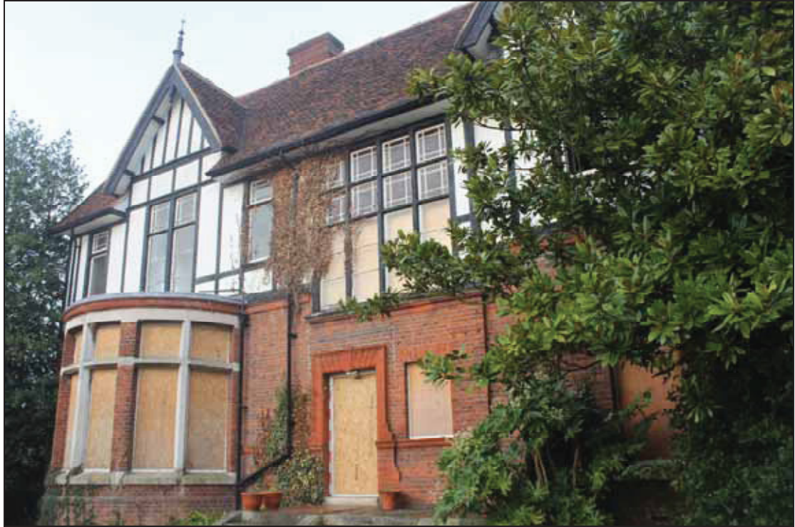
Plate 5 South-west elevation, taken from the south-east (DP 79)
