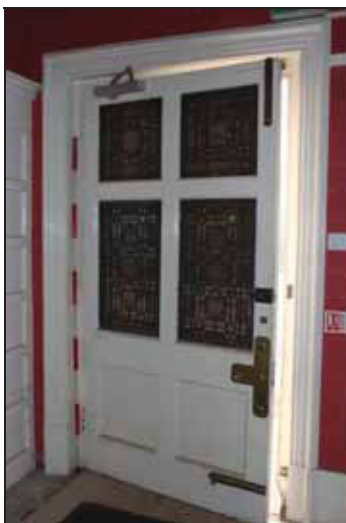
Main door with upper stained glass and lower panelling, GF01, taken from the west
