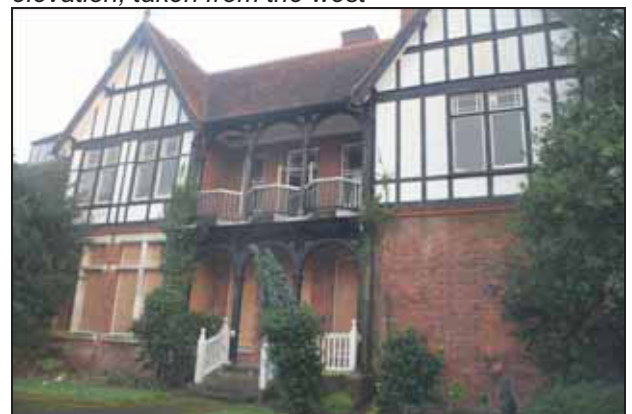
Heavy transom and mullion window with upper panels containing some stained glass, south-west elevation, taken from the west
