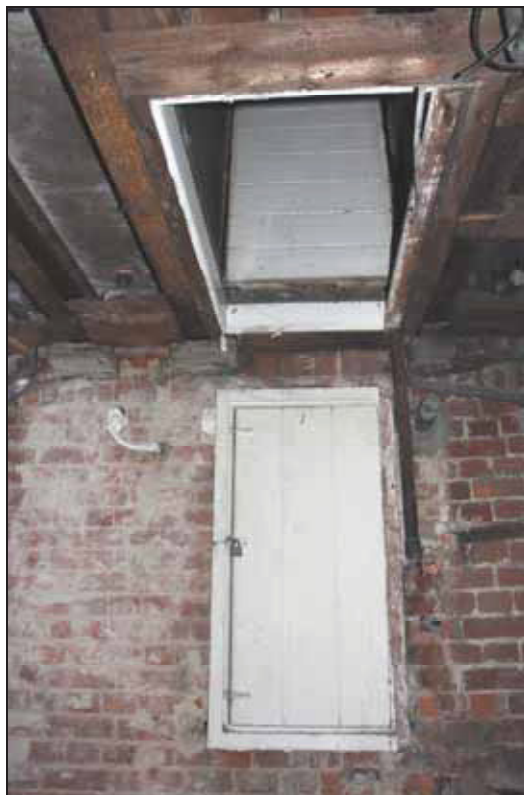
Plate 28 Small door to exterior with loft hatch above for access to water tanks, TF01, taken from the north-east (DP 303)
