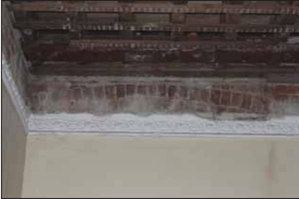
Exposed arch possibly for a large window or door now reduced to a domestic sized door, GF08, taken from the south-west
