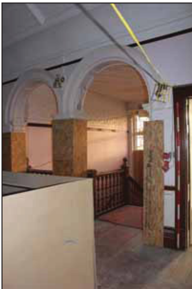
Arch supports given the decorative effect of columns, FF01, taken from the west
