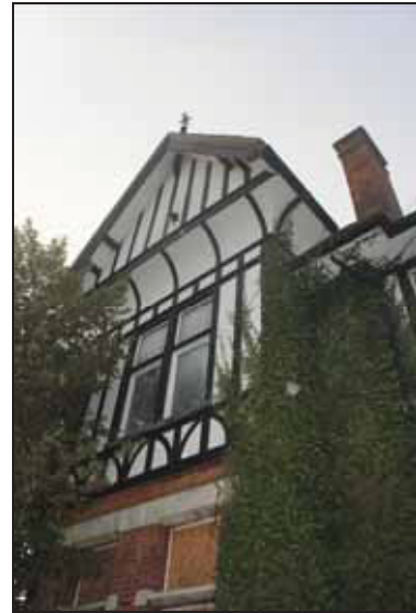
Upper decorative timber framing with jettied gable to south-east elevation, taken from the east
