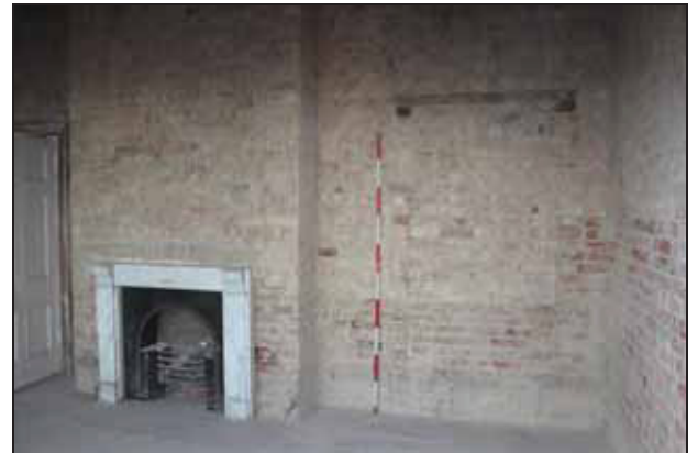
Chimney stack stripped back with removal of surround and grate, FF06, taken from the south-west
