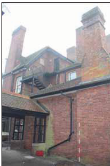
Tall chimney stack with tumbled-in brickwork, service range, north-east elevation, taken from the north
