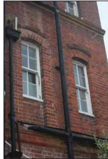
Slightly recessed sash windows beneath cambered arches, campanile, south-east elevation, taken from the south
