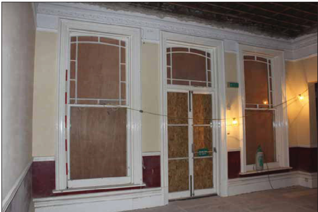
Plate 16 GF07, taken from the south-east (DP 198)
