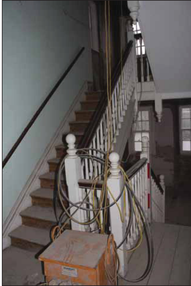
Plate 25 Back stair, FF11, taken from the west (DP 292)
