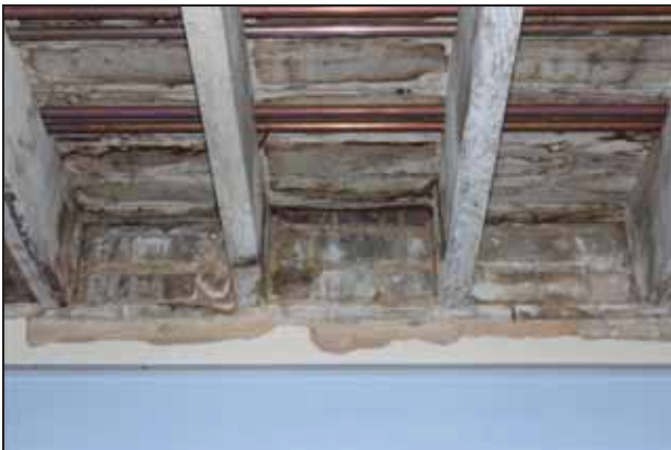
Ceiling joists set into the external wall of the north-east block, GF06, taken from the south-west
