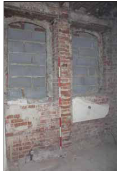
Blocked windows, ground floor of the campanile, GF18, taken from the south-west
