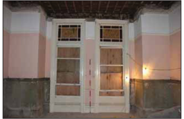
Double sashes with overlights of coloured glass, GF04, taken from the north-west
