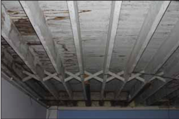
Ceiling joisting supported by cross-bracing, GF06, north-east block, taken from the south-west
