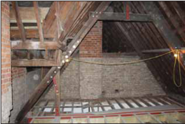
Hipped rafter arrangement surrounding central light well, SF09, taken from the south
