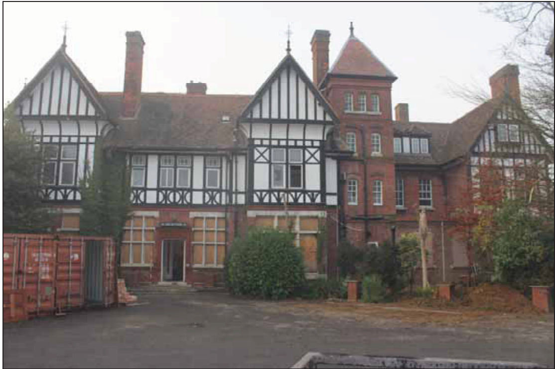
Plate 1 Pearse House, south-east elevation, taken from the south-east (DP 70)
