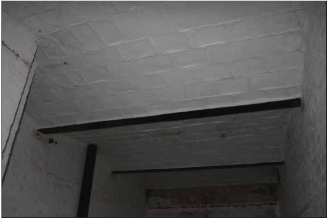
Plate 11 Jack-arch ceiling supports above BF06, taken from the south (DP 118)
