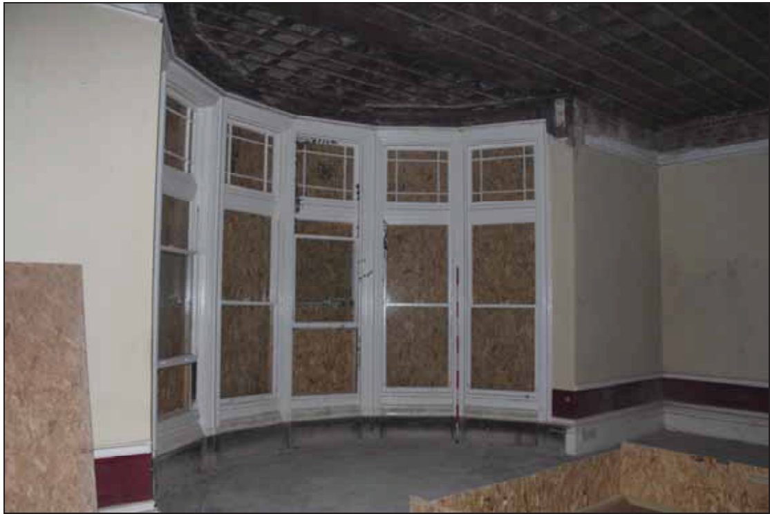
Plate 17 Large bay window, GF08, taken from the east (DP 147)
