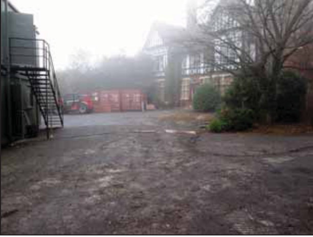
1 General shot of site before excavation
