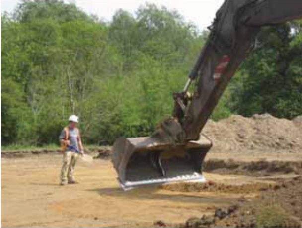
General shot. Topsoil stripping in progress. Northern corner of site, looking north.
