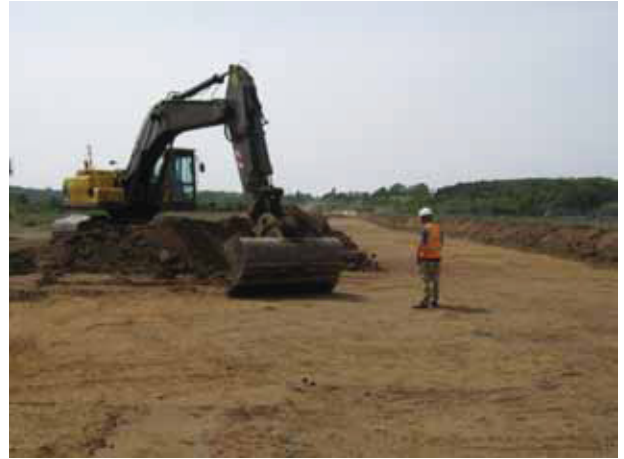
General shot. Topsoil stripping in progress. Northern end of site, looking southwest.
