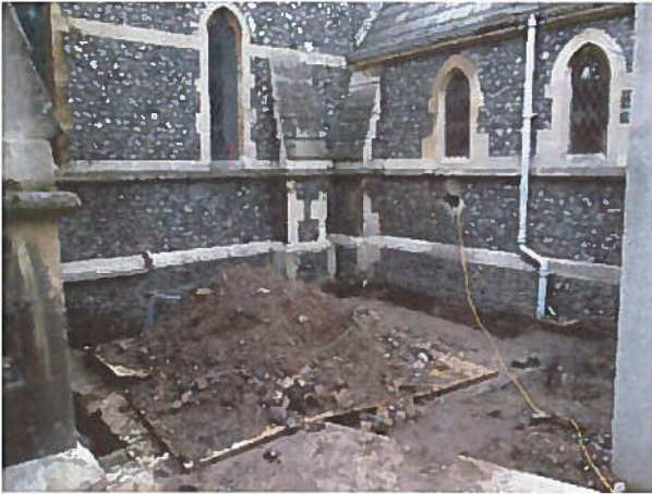
DP 1. The area of monitoring. Looking north.
