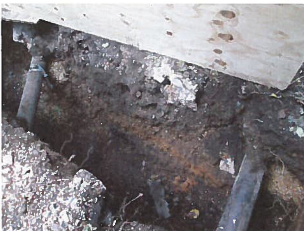
DP 5. Southern part of the area. Sample section 2. Looking north-north-east.
