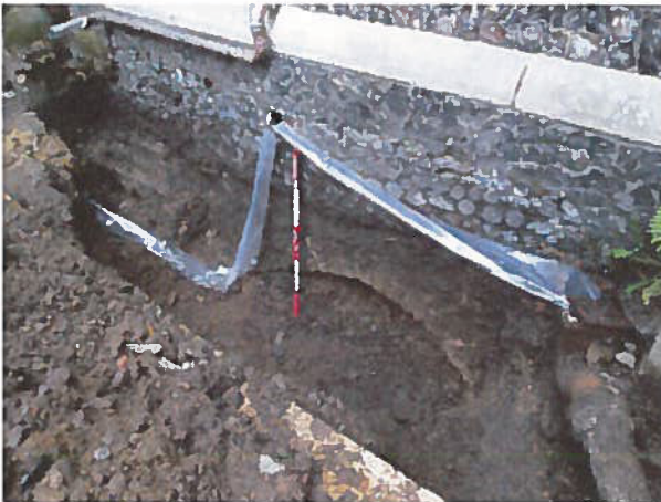
DP 3. North-western side of the area. Looking west.
