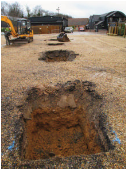
DP 3. Northern row of foundation pits. Looking east-north-east.
