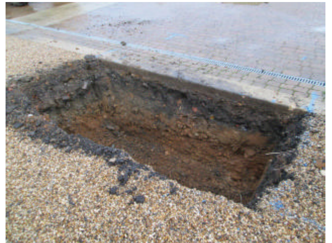
DP 10. Southern row of the pits, Pit 14. Looking east-north-east.
