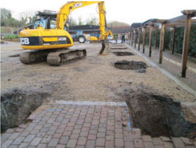
DP 9. Southern row of the pits. Looking east-north-east.
