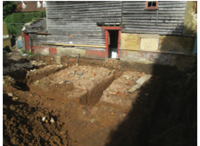
DP 2. Excavated foundation trenches. Looking north-north-west.
