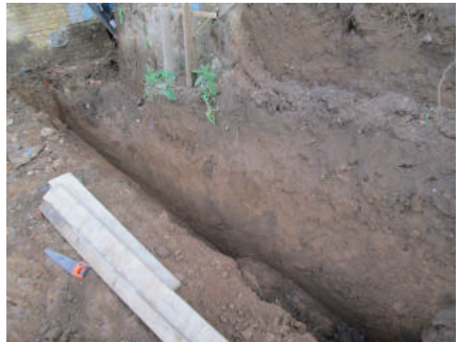
DP 4. Eastern foundation trench. Looking north-north-east.
