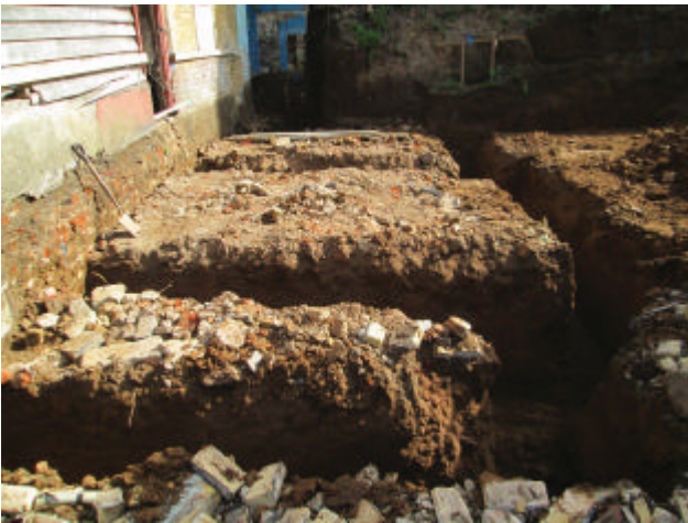
DP 3. Foundation trenches. Looking east.
